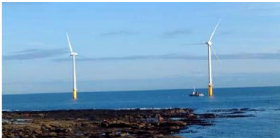
Figure E.2: Coastal Explorer laying the inter-array Cables
