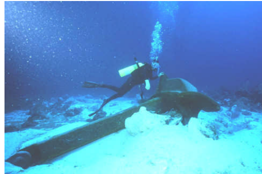
Figure A.15: Anchoring (courtesy Nexans)
