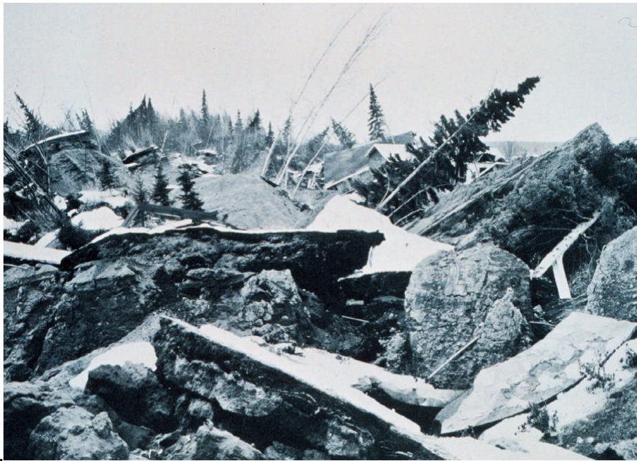
Figure 5.2: The largest landslide in Anchorage occurred along Knik Arm between Point Woronzof and Fish Creek, causing substantial damage to numerous homes in the Turnagain-By-The-Sea subdivision. [Ref. 5.5].
