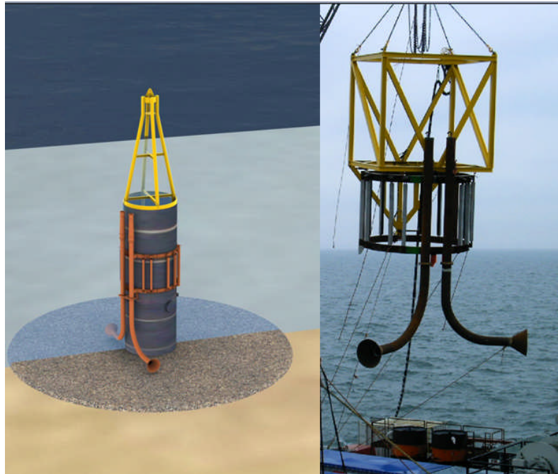
Figure 9.11: J –Tube assembly.
