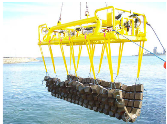
Figure 5.7: ROV deployment of concrete protection
