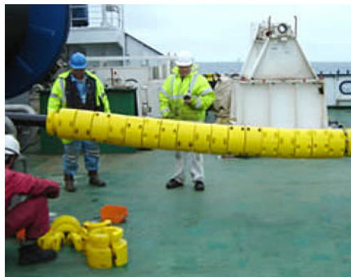
Figure 8.10: Proprietary system to protect the Export cables to London Array (Courtesy Cicor International)
