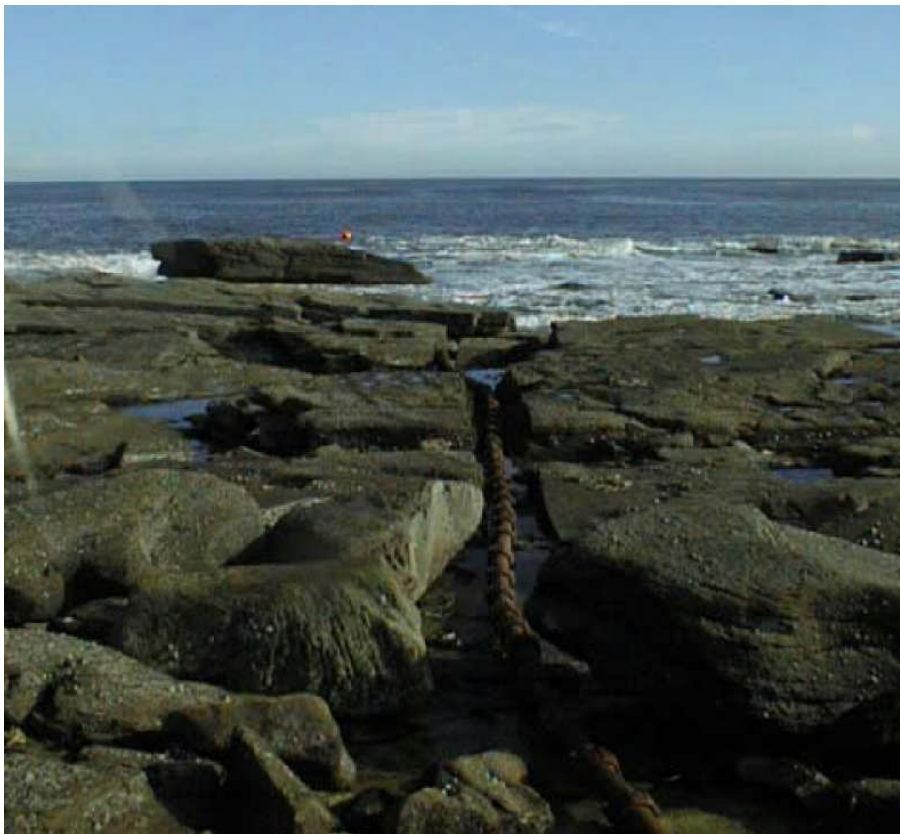
Figure E.4: Shore Connection dug into the Rocks (Source: Figure 12 www.berr.gov.uk/files/file_18014.pdf )
