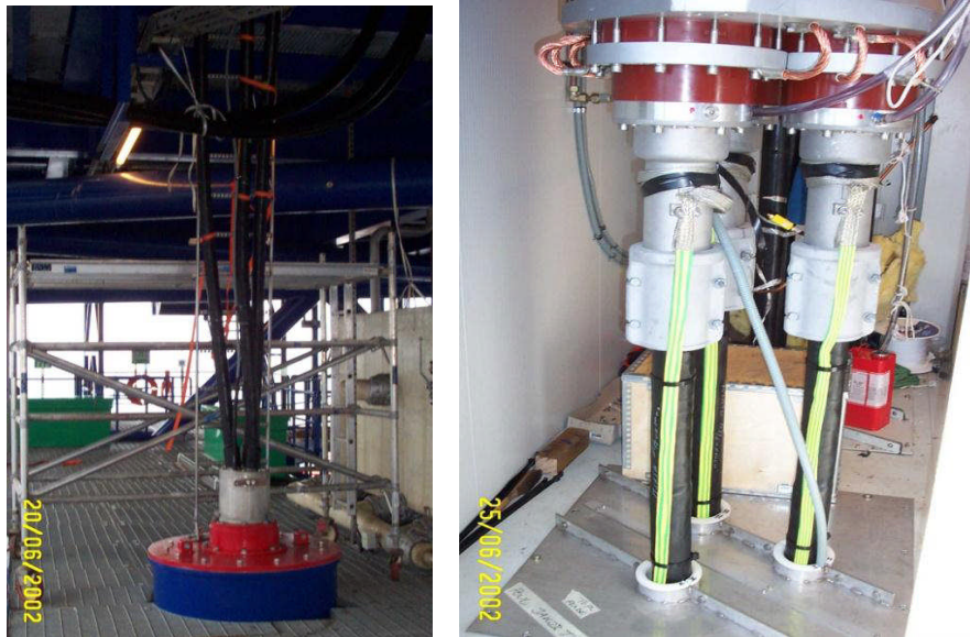
Figure 4.5: Cable Terminations at Horns Rev 2 (Courtesy Nexans)
