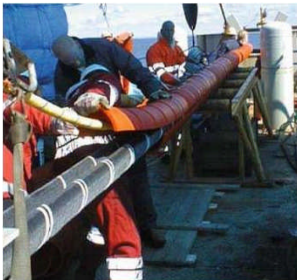
Figure D.11: Protective Plastic shells
