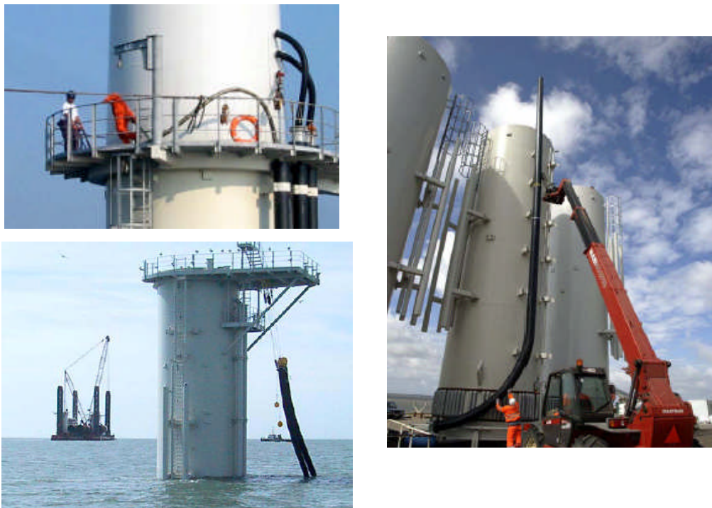
Figure 9.13: Photos of the Installation process (Source: Elsam 2002)
