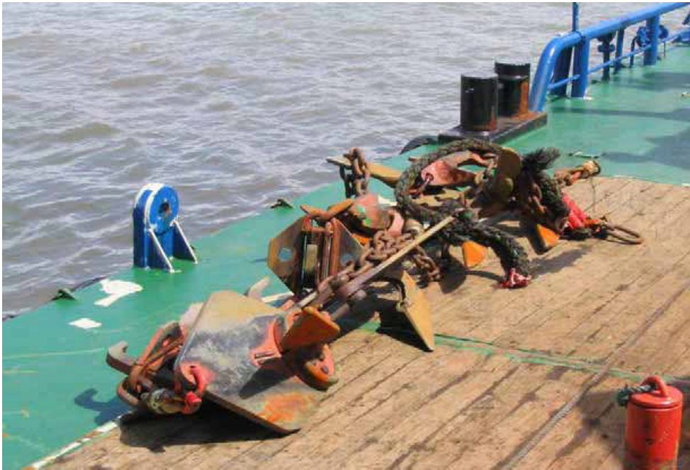
Figure A.11: Clearing debris off the seabed
