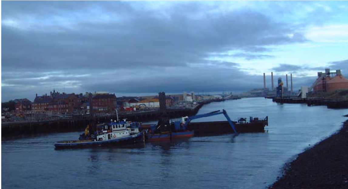
Figure E.5: Dredger Operation with Pontoon alongside.
