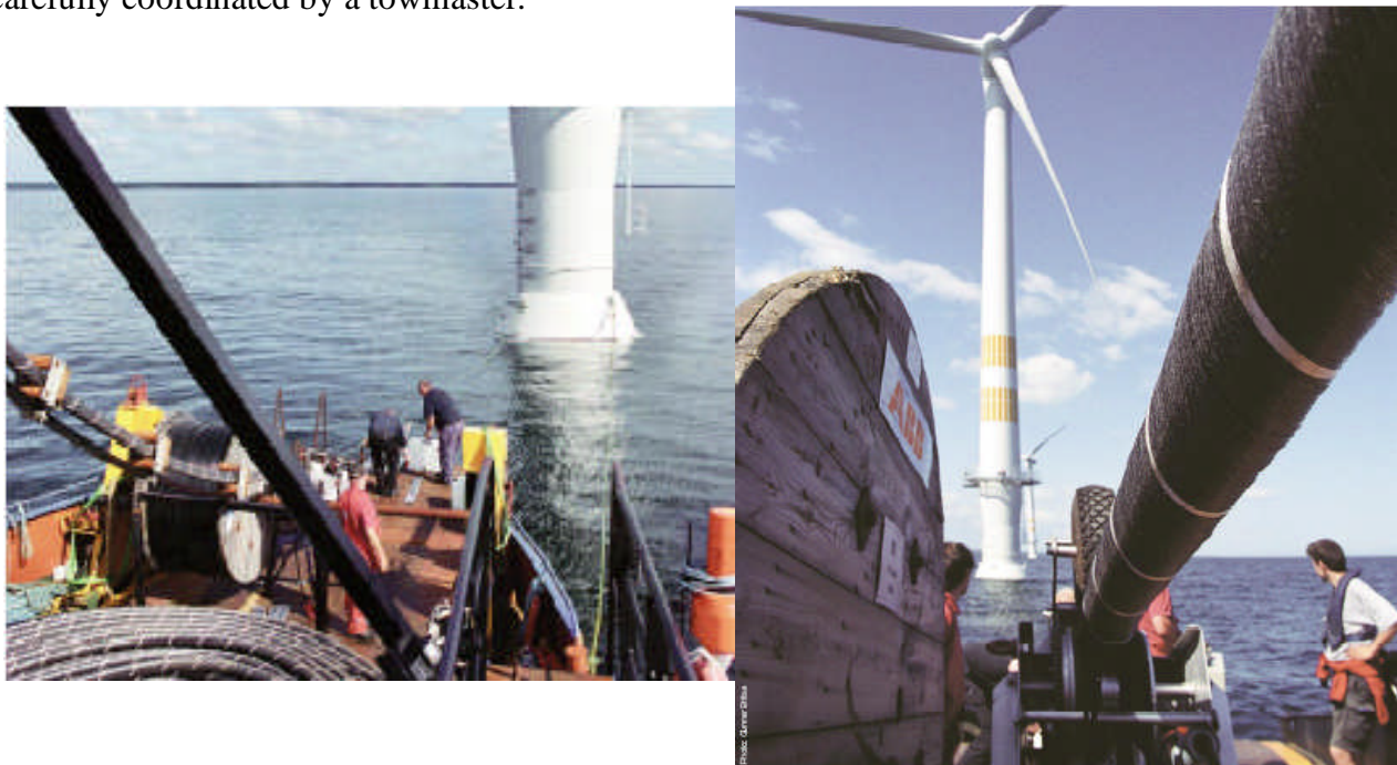
Figure D.12: Installation Vessel installing the cable (Courtesy ABB).
