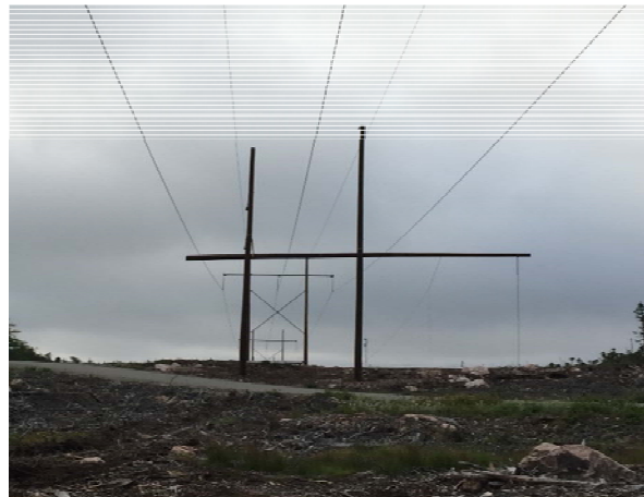
Photo 20 - HVAC line near Granite Canal – Pictures show rider poles used for stringing over roads
