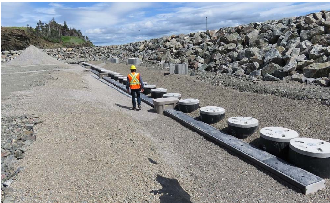
Photo 7 - Indian Head Grounding Site – View inside of rock berm (electro yard) showing row of 40 grounding wells awaiting installation of grounding electrodes, with adjacent cable duct.
