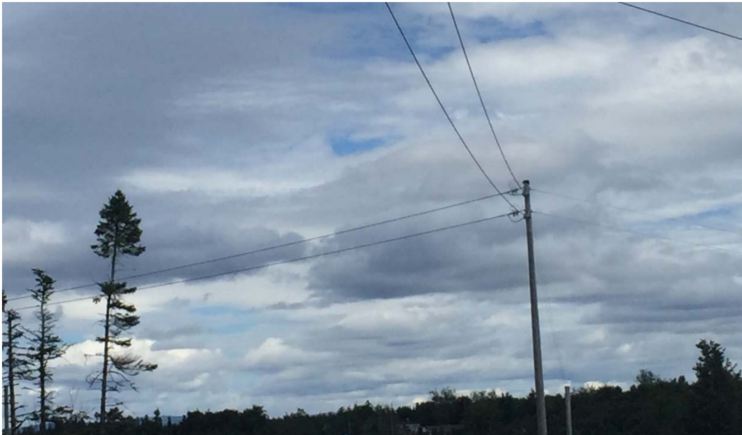
Photo 4 - Close picture for the strung grounding line – Sample dead-end structure
