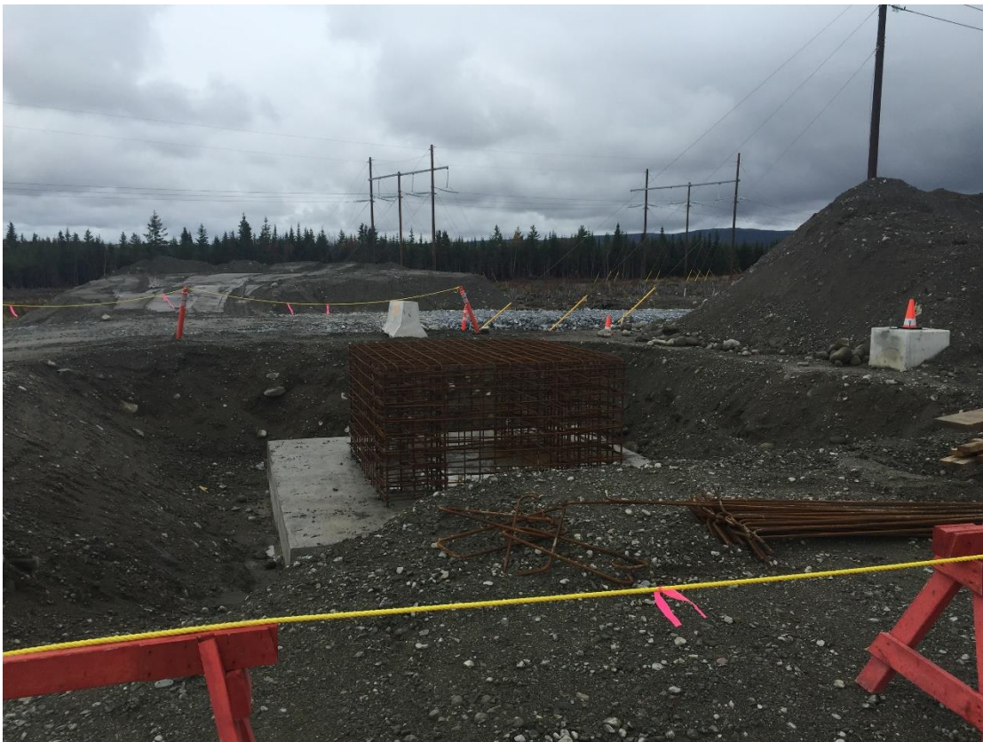
Photo 8 - Bottom Brook – Foundation work for lightning tower.
