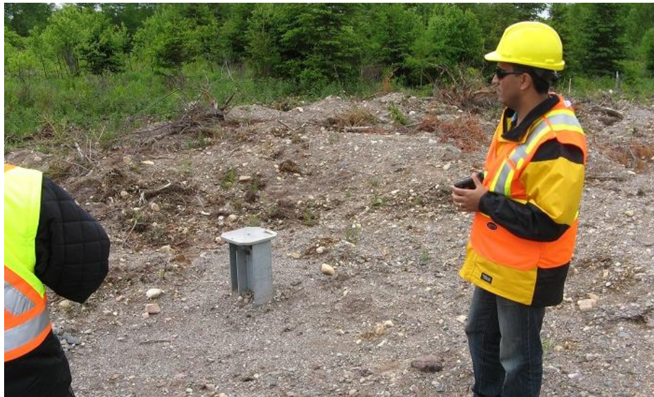
Photo 19 - Pin footing for tower 144.
