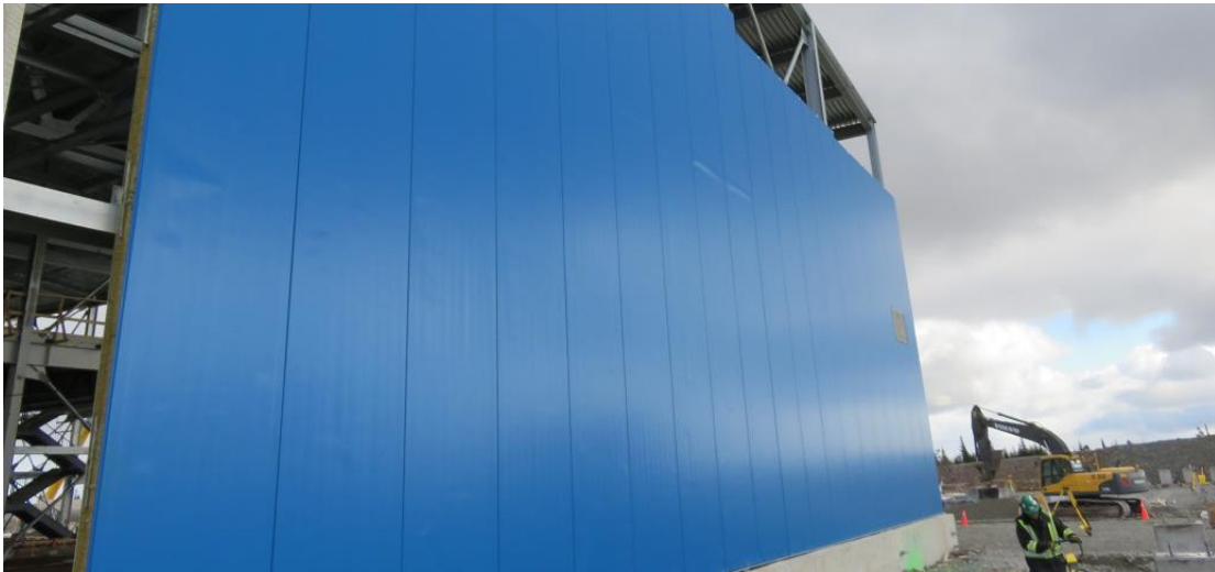
Photo 29 - Woodbine – close-up view of installed wall cladding showing several surficial buckled zones. This cladding was to be removed and replaced.
