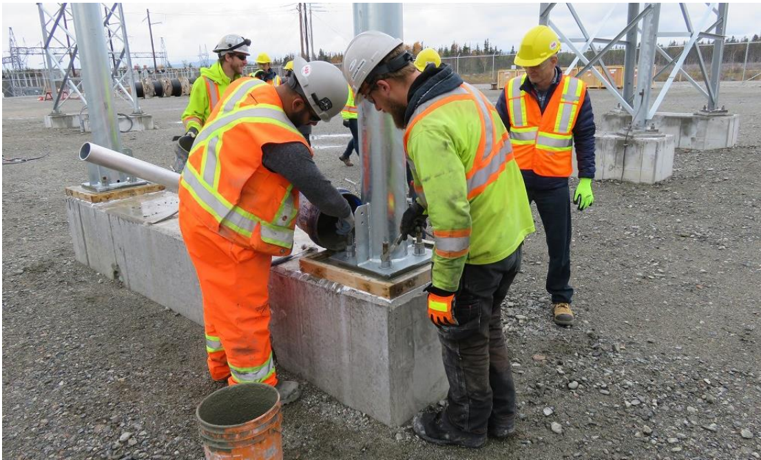
Photo 7 - Bottom Brook – grouting the base of a recently-installed steel structure.
