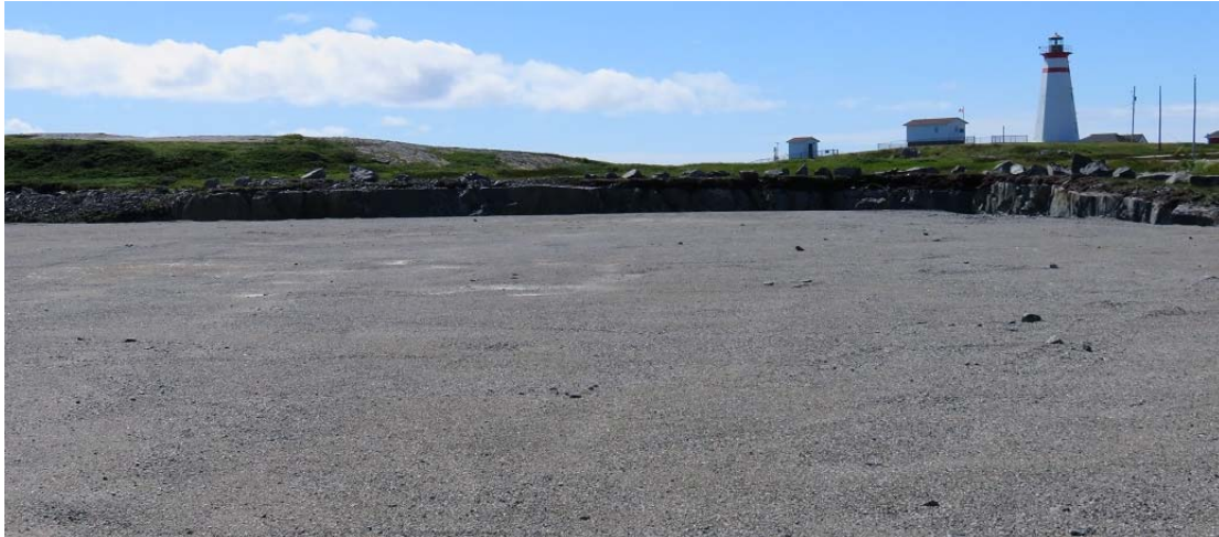
Photo 8 - Cape Ray landfall site – HDD drill pad.
