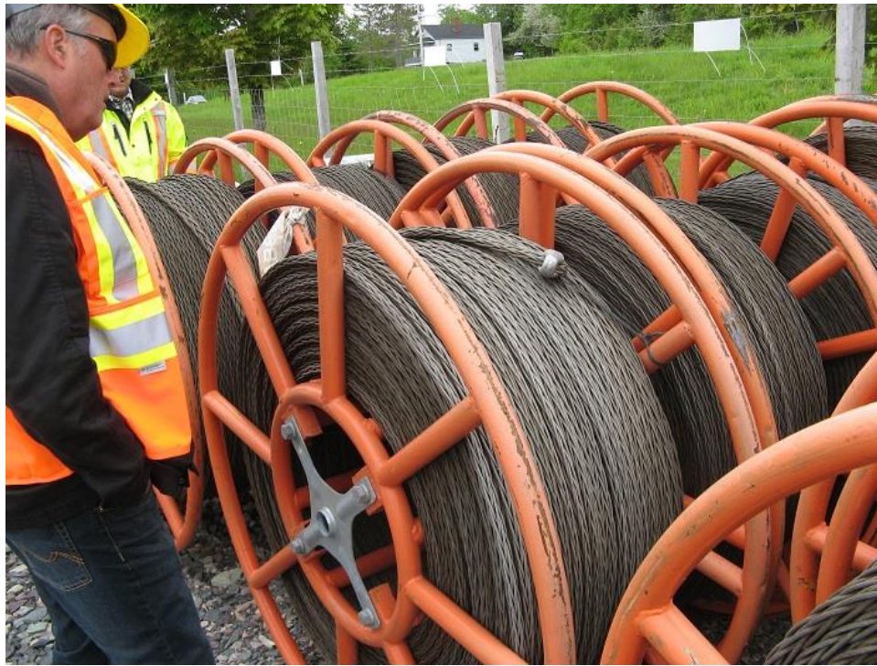
Photo 8 - Guy wire for towers.
