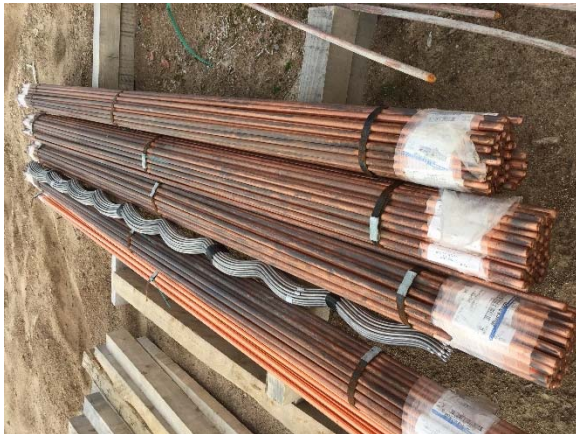
Photo 24 - HVAC line near Granite Canal – Picture on the left shows some of the materials (grounding rods and armor rods) and the picture on the right shows the vibration dampers.
