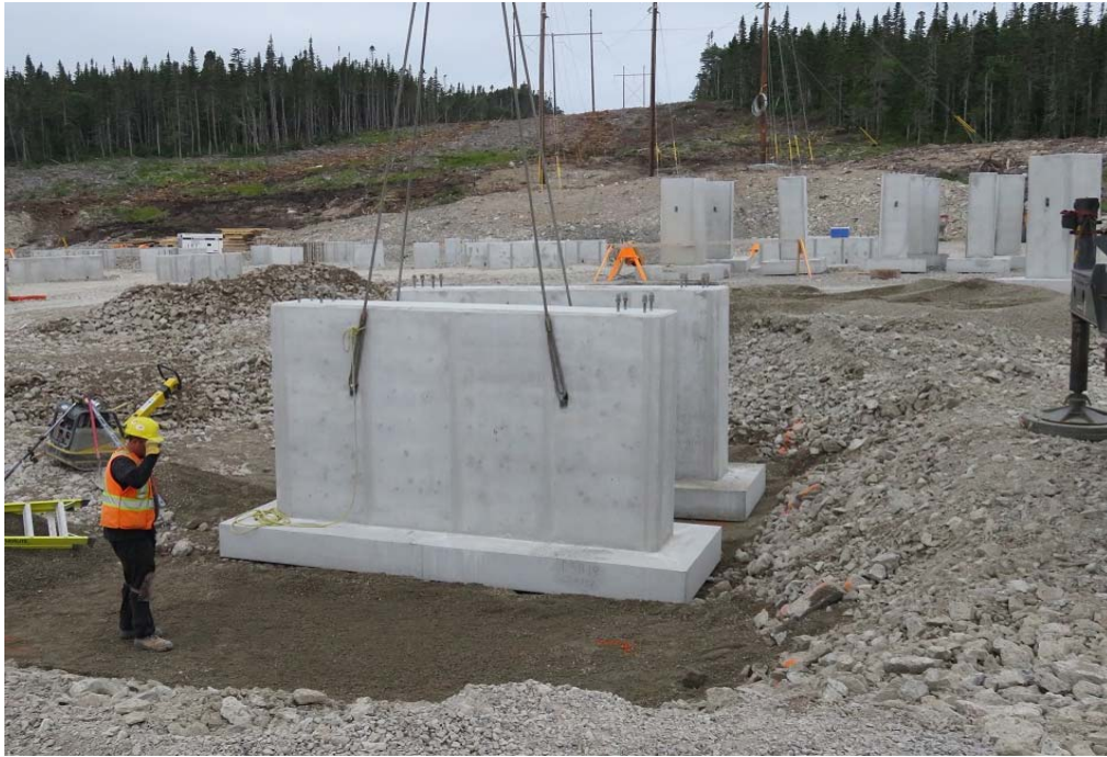
Photo 29 - Granite Canal Switchyard – mobile crane placing precast concrete footing on prepared sub-base.
