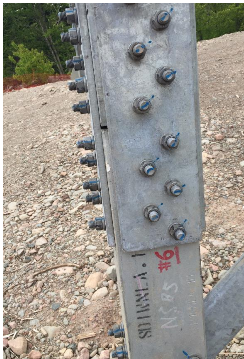
Photo 20 - Marking to confirm the bolt torque
