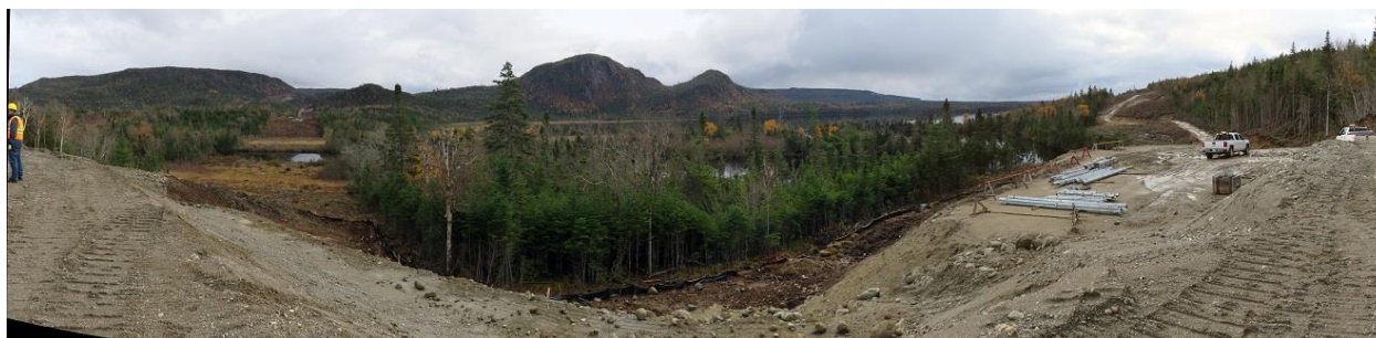
Photo 9 - HVDC line – panorama view of HVDC right of way from site SA7. Right-of-way crosses Bottom Brook at left. Steel for tower mobilized to site at right.
