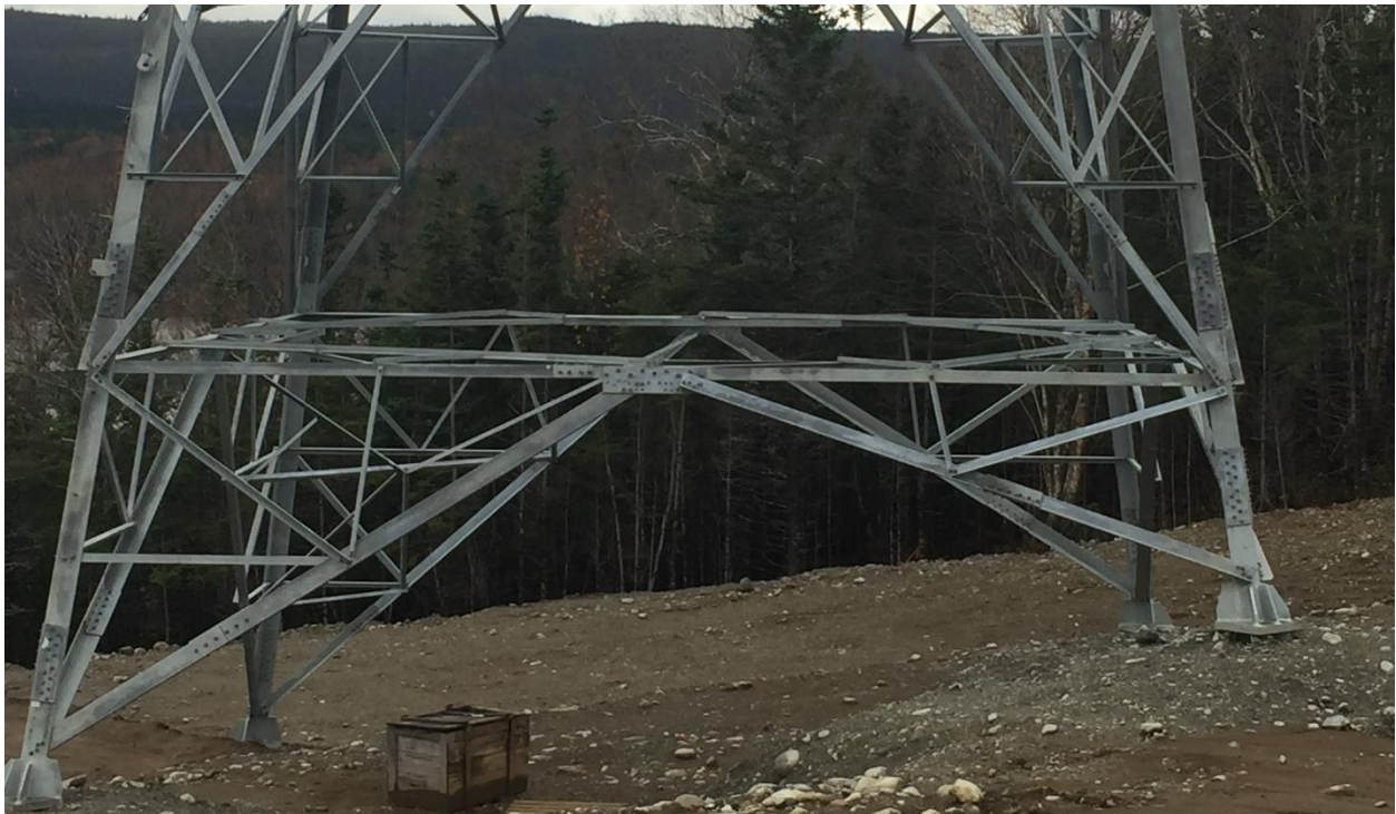
Photo 15 - HVDC – Erected lattice structure tower
