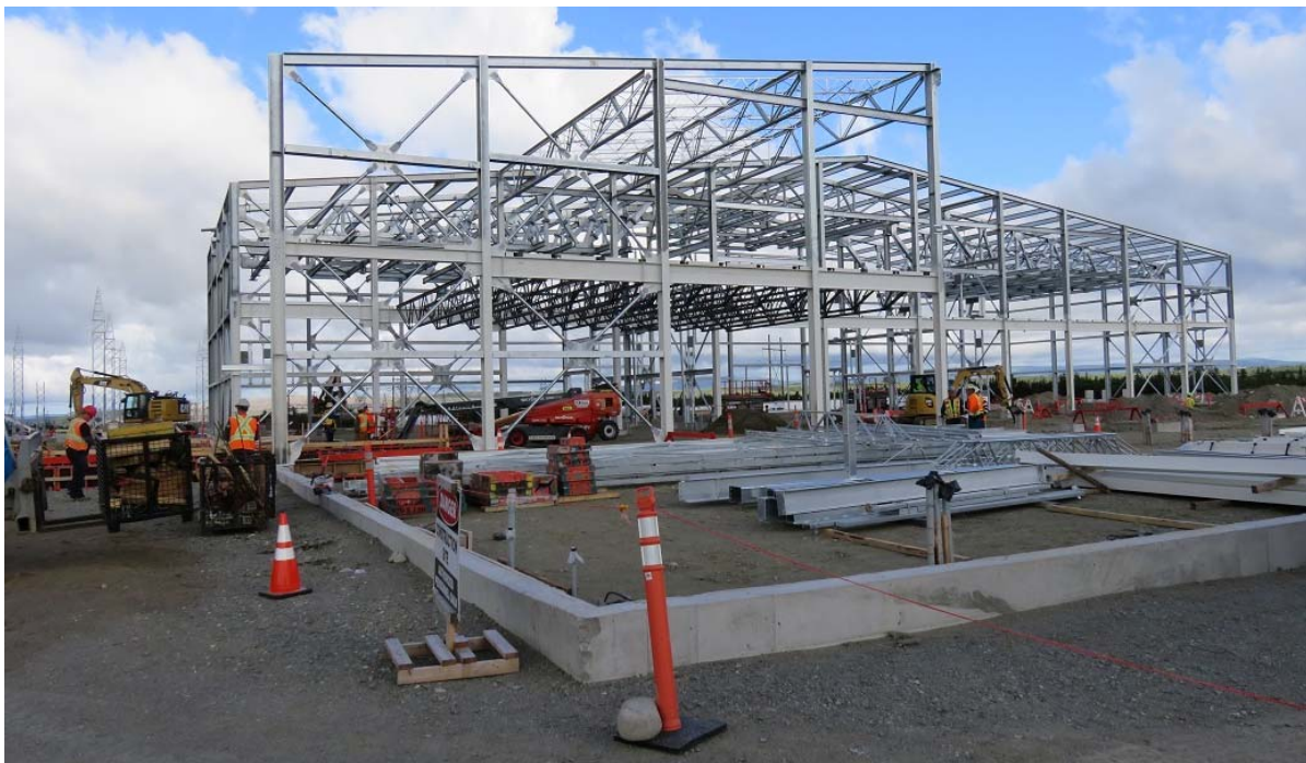
Photo 13 - Bottom Brook – partially-erected steel frame for converter building. The concrete foundation in foreground indicates the full extent of the building when it is completed.
