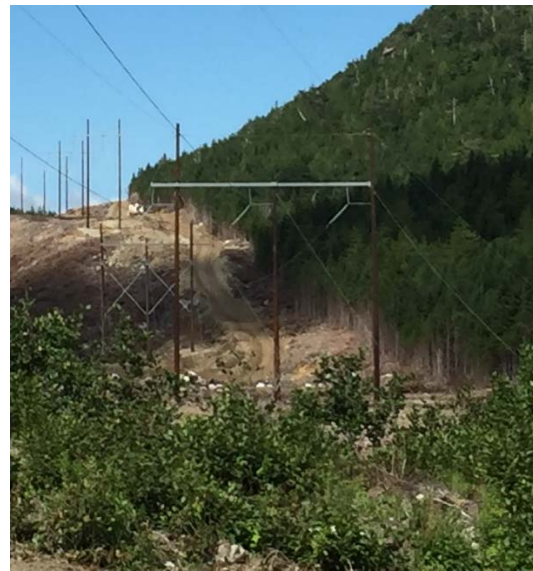
Photo 18 - HVAC line at crossing of Southwest Brook along Burgeo Highway, with three-pole angle structures in foreground and two-pole structures in background.
