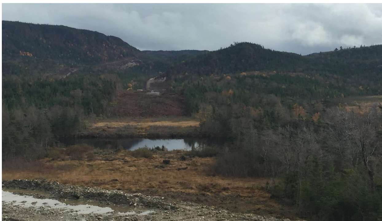
Photo 10 - HVDC line – Right of way clearing
