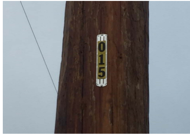
Photo 23 - HVAC line near Granite Canal – Picture on the left shows the pole tag (80-1 or 80 feet Class 1) and the picture on the right shows typical structure number tag.
