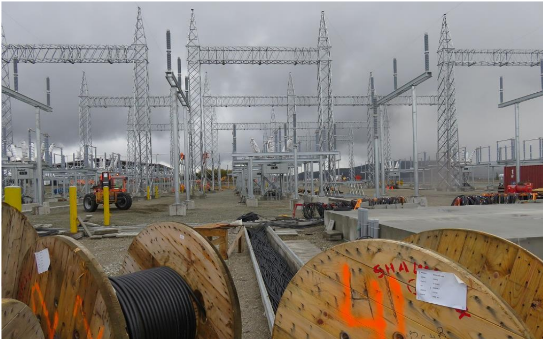
Photo 5 - Bottom Brook – general view of completed structural steel in substation with cable duct in foreground.
