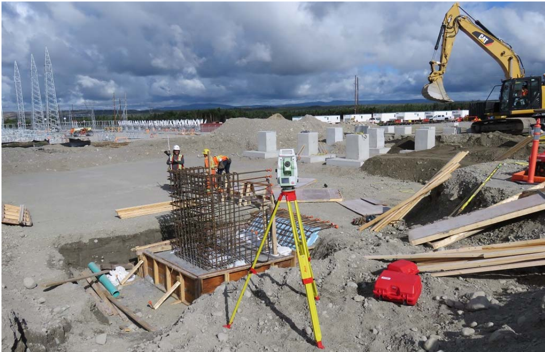
Photo 16 - Bottom Brook – General view of a cast-in-place concrete equipment footing in foreground, with closely-spaced precast concrete footings being installed in centre right of photo. Note the safetycaps on exposed horizontal rebar ends.
