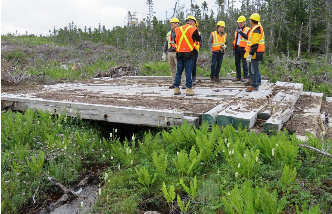
Photo 27 - HVAC line near Granite Canal – typical crossing of small watercourse using timber mats.
