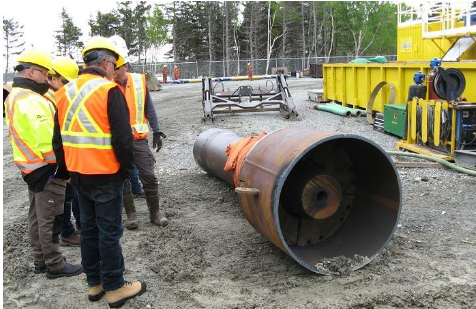
Photo 4 - Casing hammer used to drive 42-inch casing.
