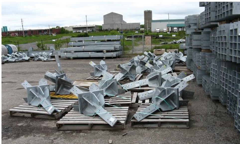
Photo 11 - Grillage footing components.
