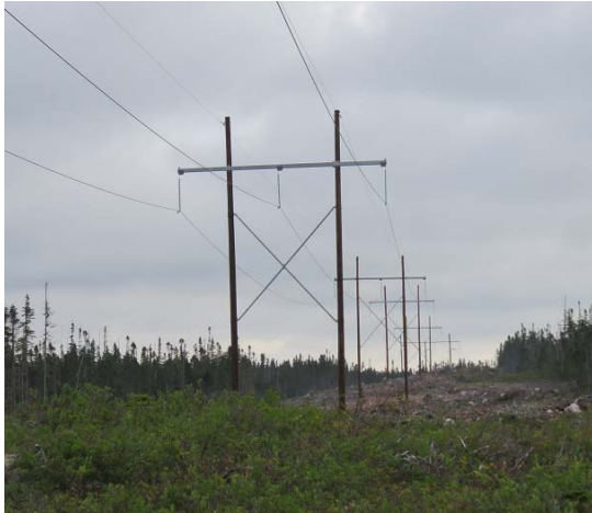
Photo 19 - HVAC line near Granite Canal – completed section of line at left, and poles with pulleys in place, ready for line stringing at right.
