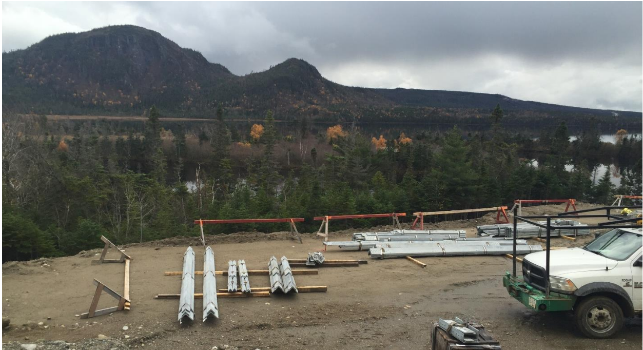
Photo 14 - HVDC – Structural members ready for tower assembly
