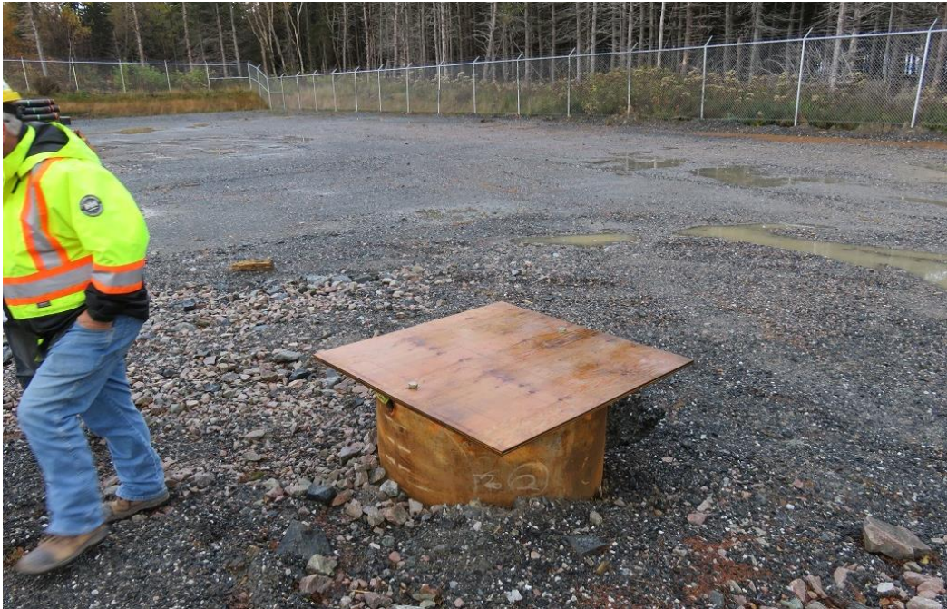
Photo 19 - Point Aconi landfall site – temporary protective cover over HDD drill hole.
