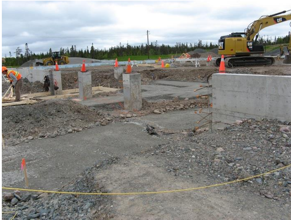
Photo 27 - Converter station foundation.
