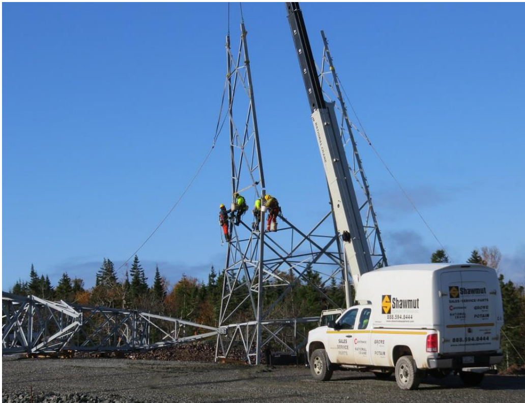
Photo 26 - Cape Breton HVDC line – tower erection in progress adjacent to Woodbine converter station site.
