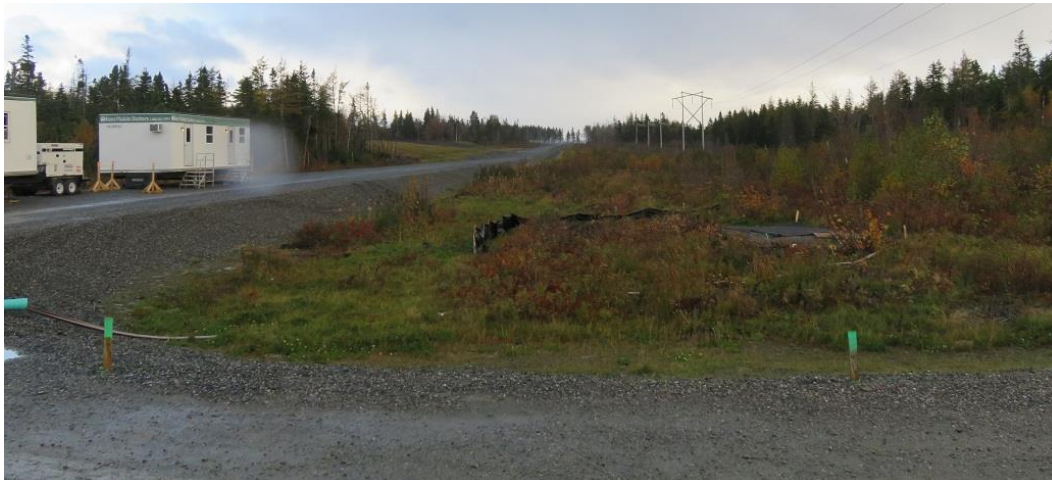
Photo 20 - View from transition compound site towards Point Aconi landfall. Underground HVDC cables will be installed along side of road.
