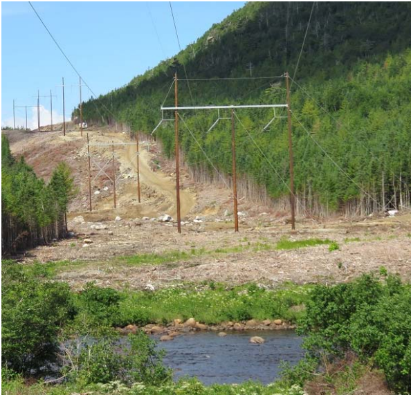
Photo 18 - HVAC line at crossing of Southwest Brook along Burgeo Highway, with three-pole angle structures in foreground and two-pole structures in background.
