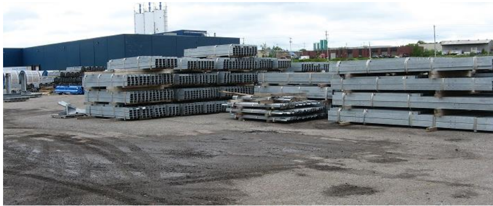
Photo 10 - Grillage and tower steel.
