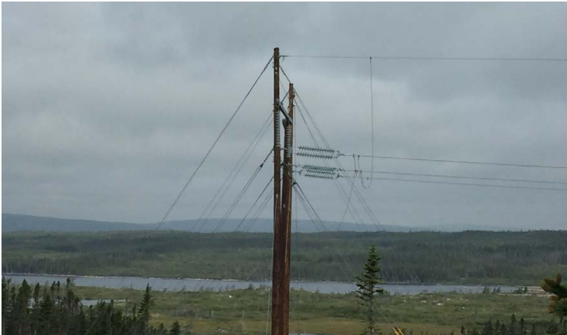
Photo 25 - HVAC line near Granite Canal – End of stringing section applying grounds.
