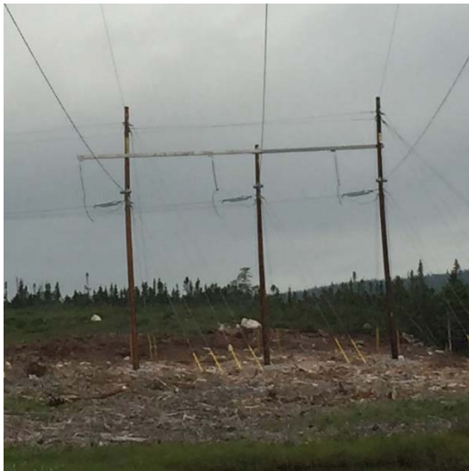
Photo 22 - HVAC line near Granite Canal – typical wood pole tangent structure (to the right) and dead-end structure to the left
