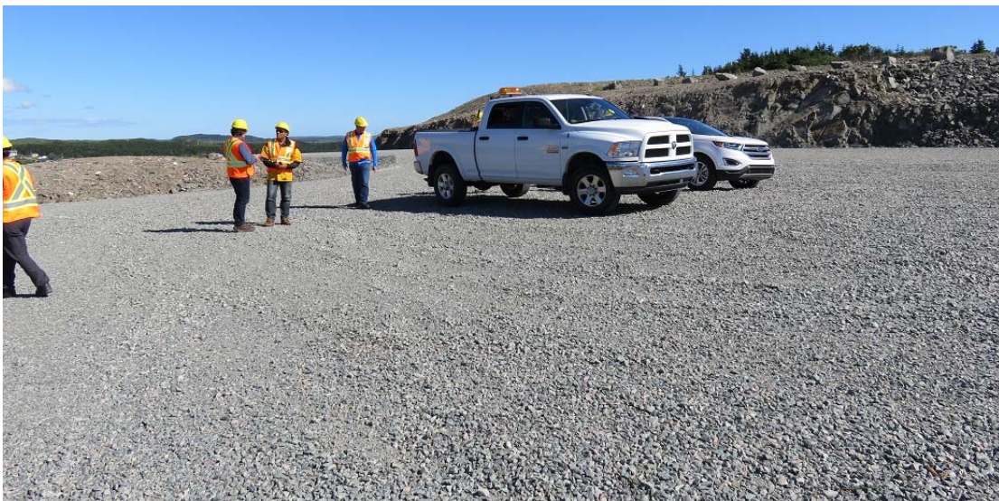
Photo 11 - Cape Ray transition compound – view looking across compound site towards access road.
