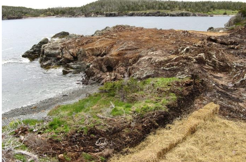
Photo 32 - Access road alignment adjacent to water area where rockfill berm will be constructed.
