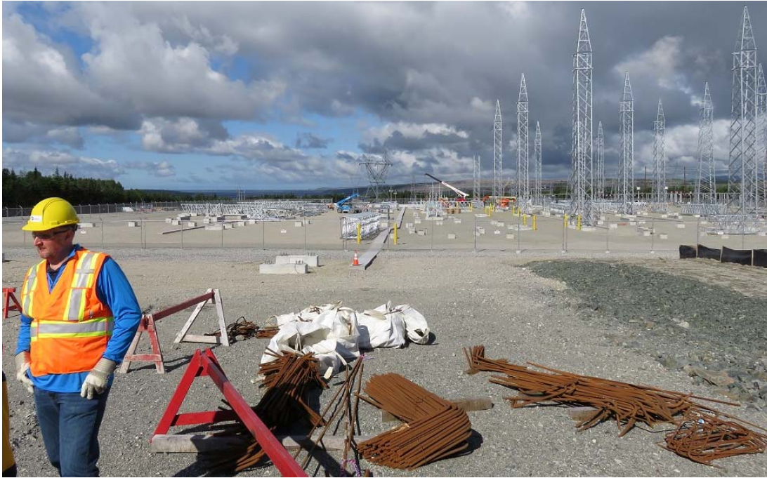
Photo 14 - Bottom Brook – switchyard construction in progress, with recently erected steel structures at right and other assembled structures laying on the ground awaiting erection at left.
