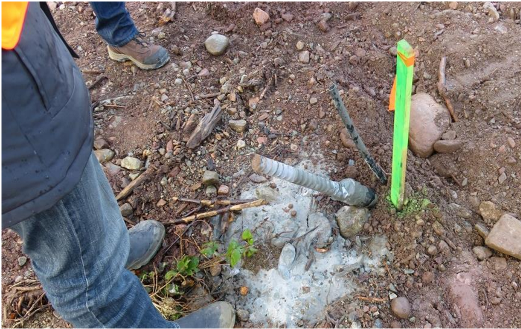
Photo 25 - Cape Breton HVDC line – typical grouted thread bar foundation anchor for guyed tower.
