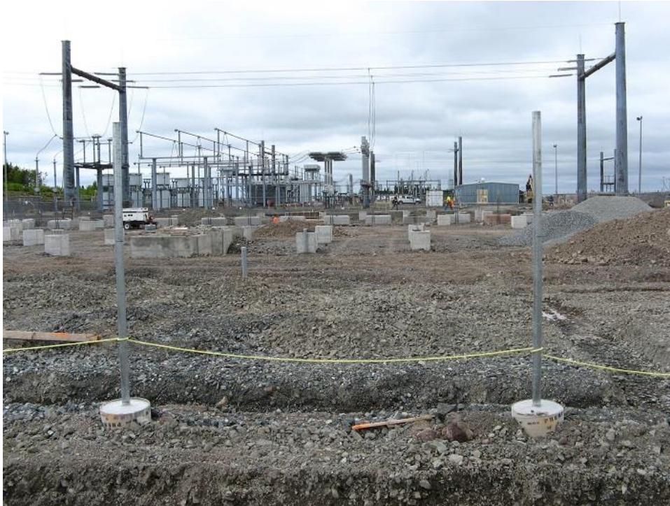
Photo 23 - Expansion of existing AC switchyard. Most of the concrete footings in foreground are precast.
