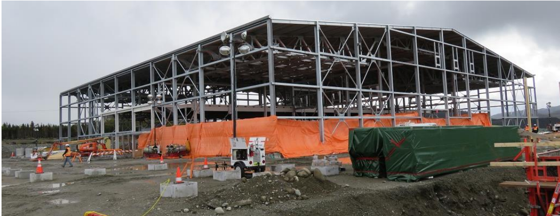
Photo 1 - Bottom Brook –steel frame of converter building.
