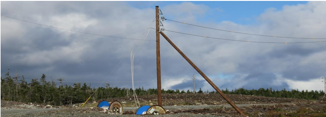
Photo 34 - Big Lorraine grounding site – panorama view inside protective rock berm. Caissons for ground rods are installed below gravel in area behind figures in centre of photo.
