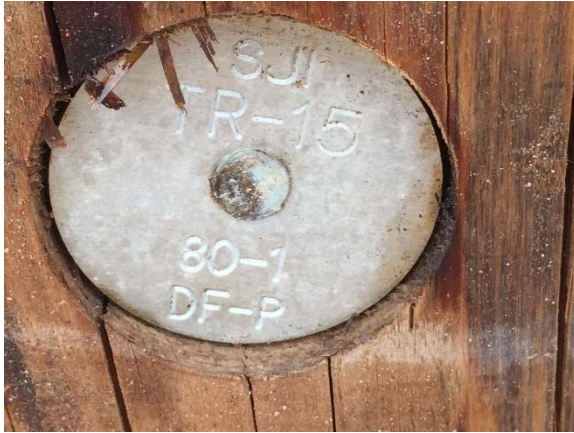
Photo 23 - HVAC line near Granite Canal – Picture on the left shows the pole tag (80-1 or 80 feet Class 1) and the picture on the right shows typical structure number tag.
