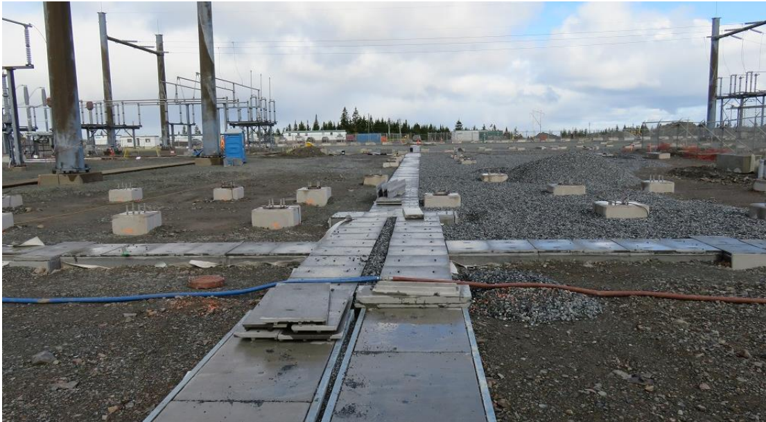
Photo 31 - Woodbine – view along cable ducts in AC substation , with numerous precast concrete footings installed and ready for structural steel and equipment installation.
