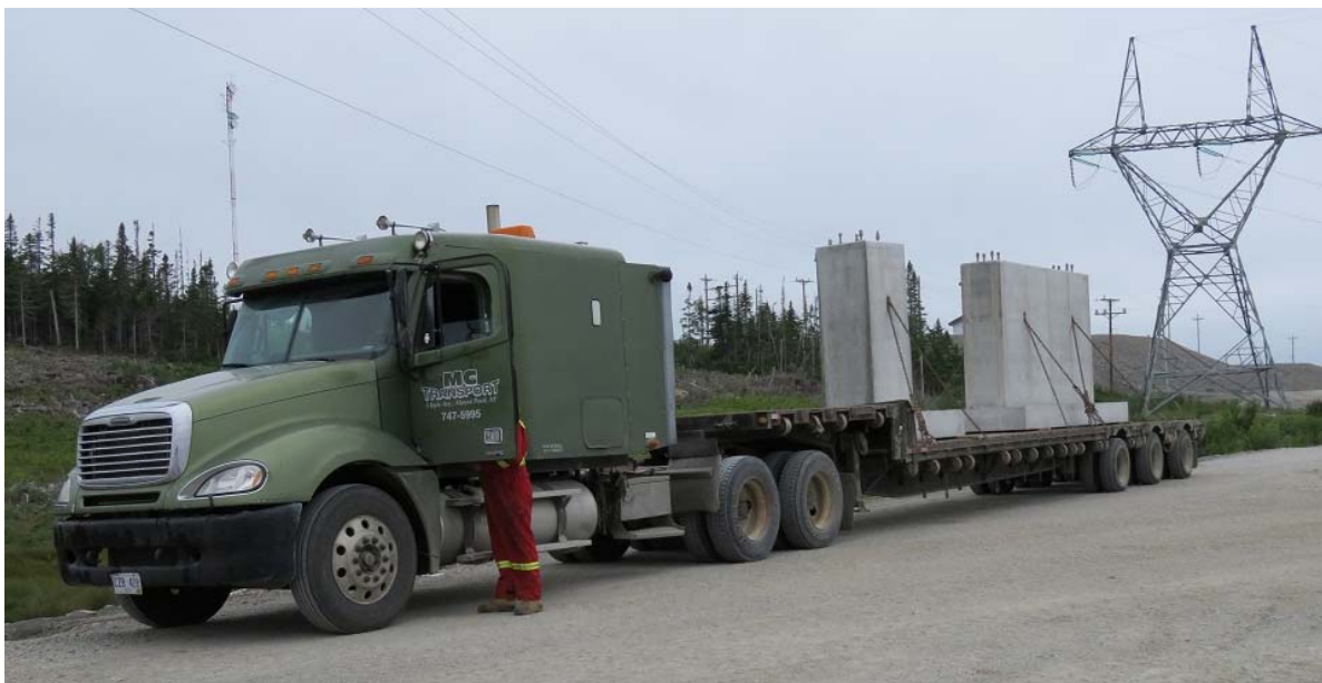
Photo 28 - Granite Canal Switchyard – two precast concrete footings being delivered from St. John's.
