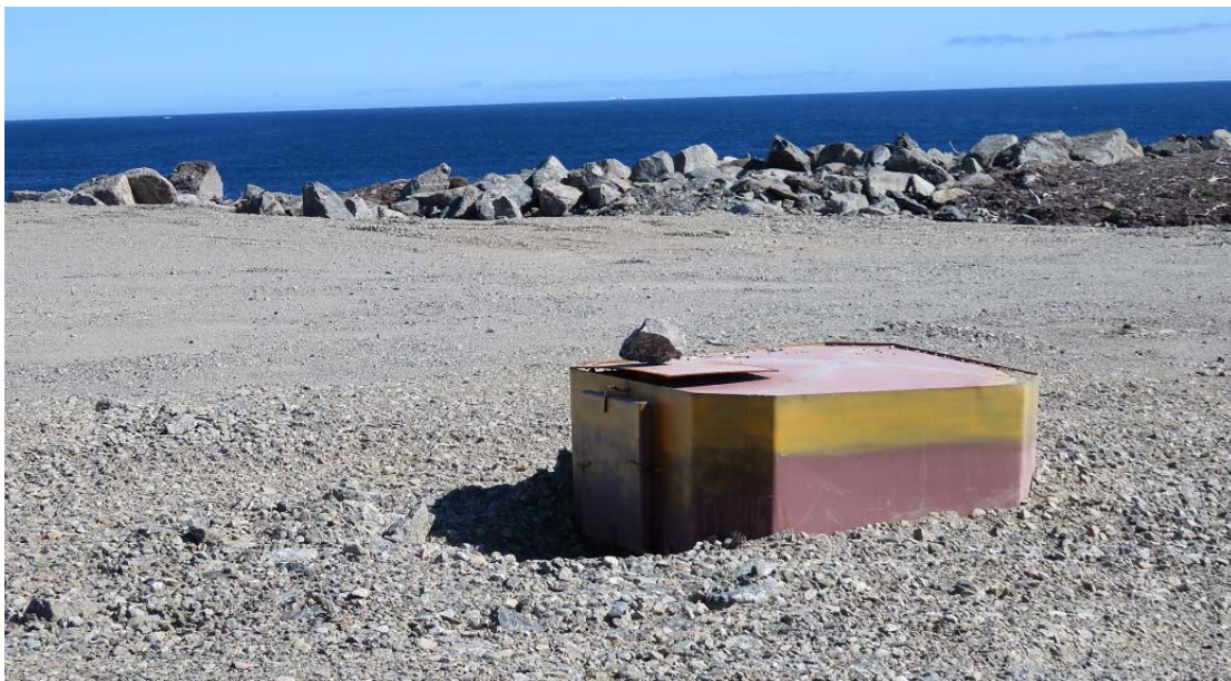
Photo 9 - Cape Ray landfall site – temporary protective cover on one of the two HDD hole collars.
