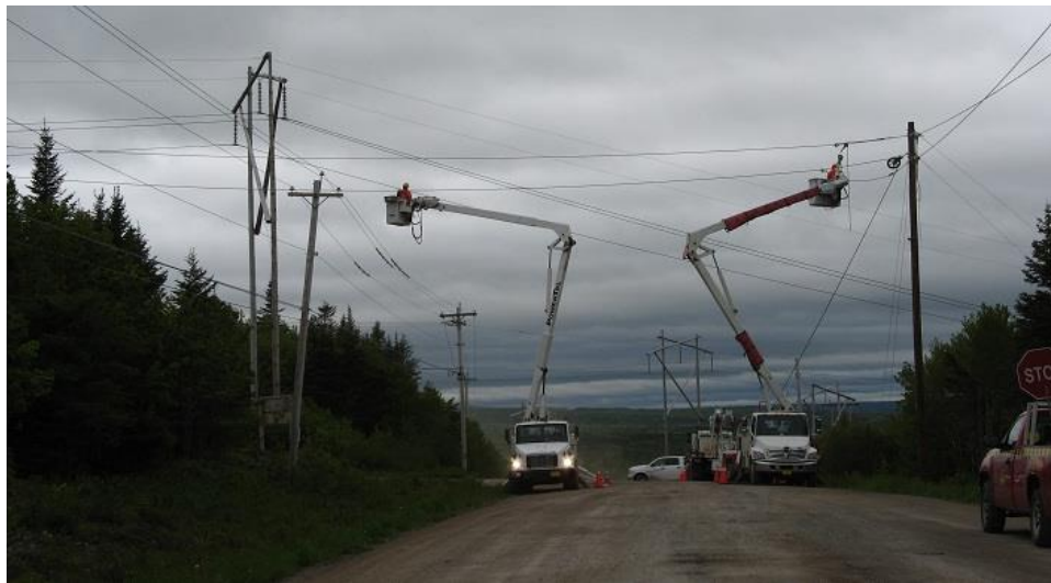
Photo 28 - Stringing grounding line across road near entrance to Woodbine converter station (PowerTel is contractor)
