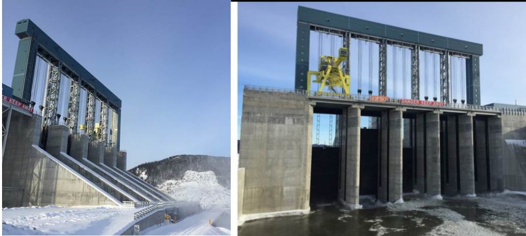
L-R: Spillway downstream and upstream at the Muskrat Falls generation facility
