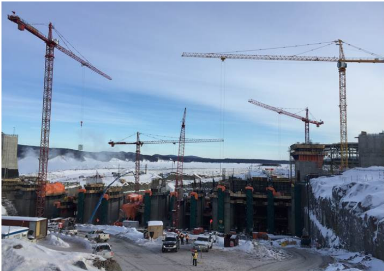
Ongoing construction by Astaldi of the Muskrat Falls powerhouse
