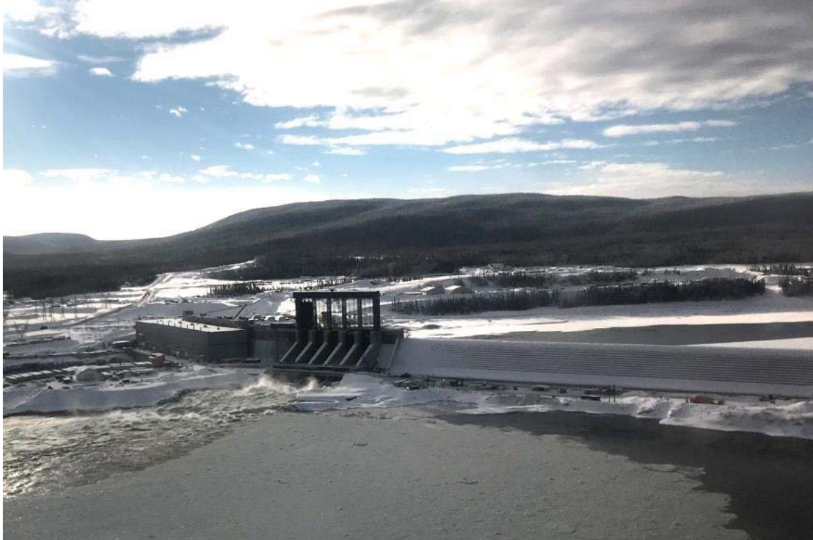
View looking upstream at the Muskrat Falls generating facility
