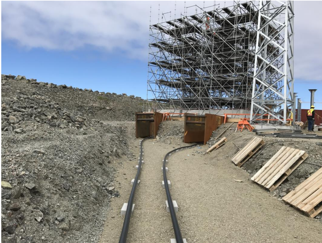
Photo 29: Scaffolding erected for land cables termination installation at the transition compound.
