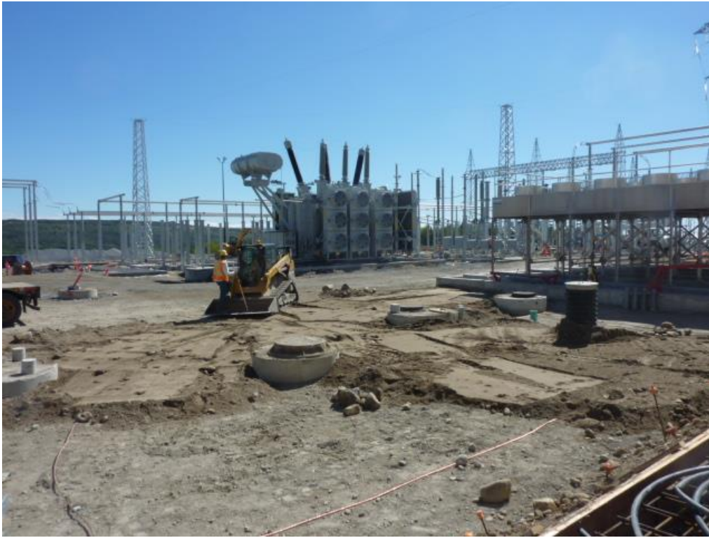
Photo 51: Woodbine converter transformer.
