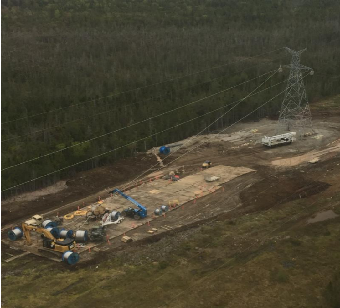
Photo 6. Stringing site / DC line.
