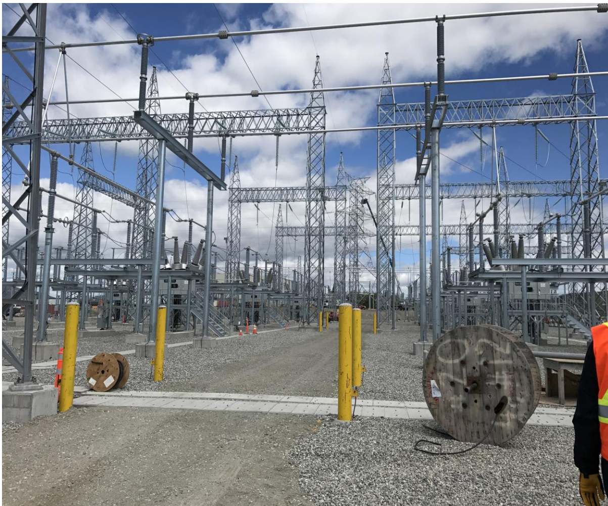
Photo 31: AC Substation nearing completion.
