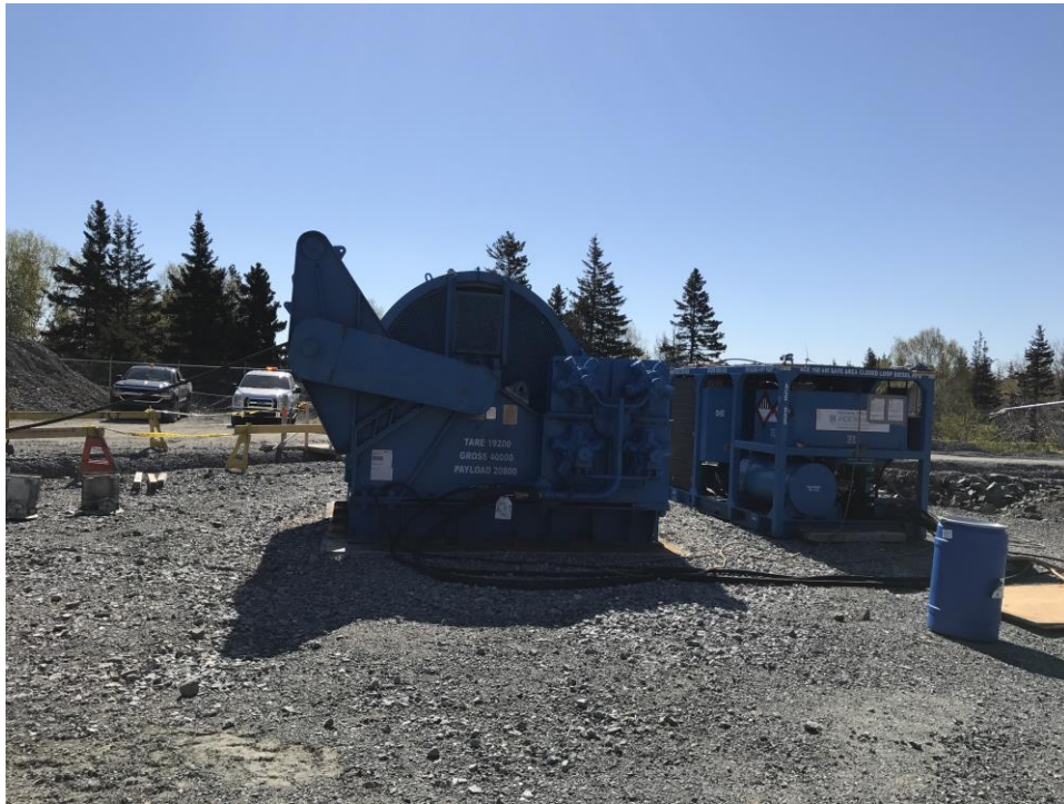
Photo 40: Winch used for pull-in subsea cables through HDD casing.
