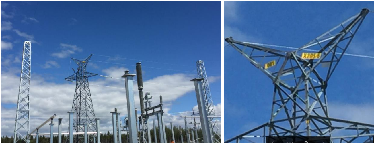
Photos 10/11. Lightning Towers and the first DC corner structure outside Bottom Brook.
