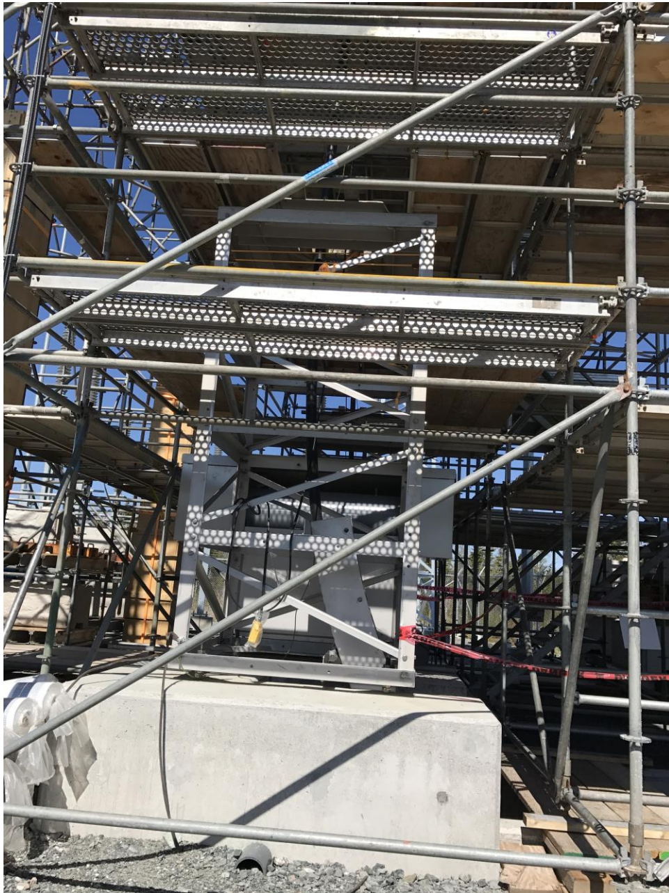
Photo 44: Scaffolding erected for land cables termination installation at the transition compound.
