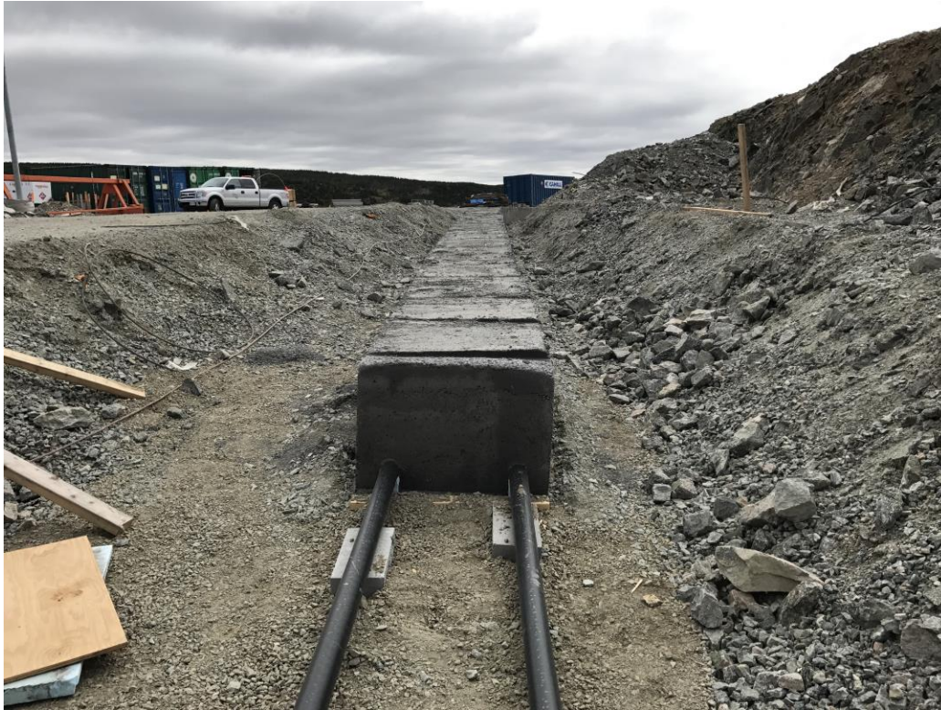
Photo 28: Land cables laid in trench and encased in protective thermal concrete.
