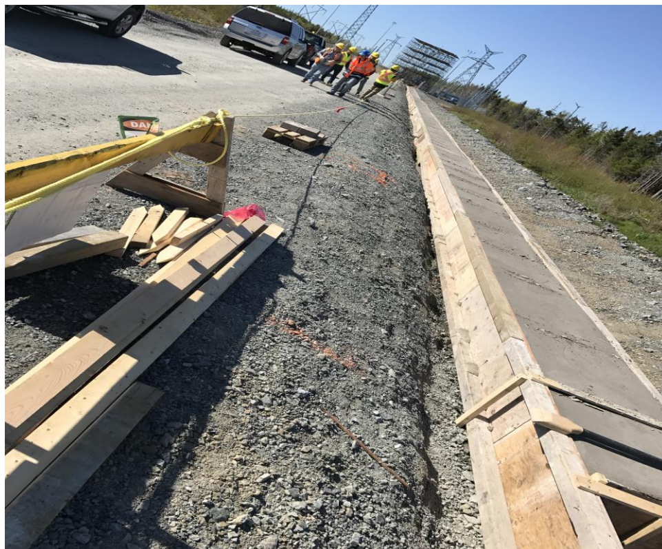
Photo 43: Land cables already encased in protective thermal concrete.
