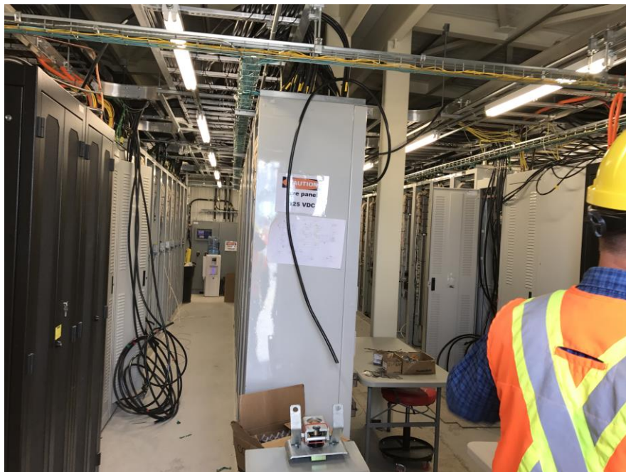
Photo 33: AC Substation Control building – ongoing cable termination.
