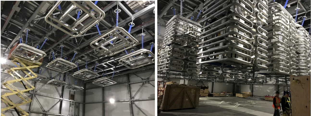
Photos 48 & 49: Converter Station - Valve Rooms at different stages of valves installation.
