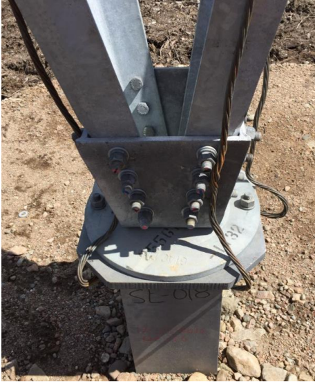
Photos 14/15. Leg Grounding / Damaged (stolen) ground wire.
