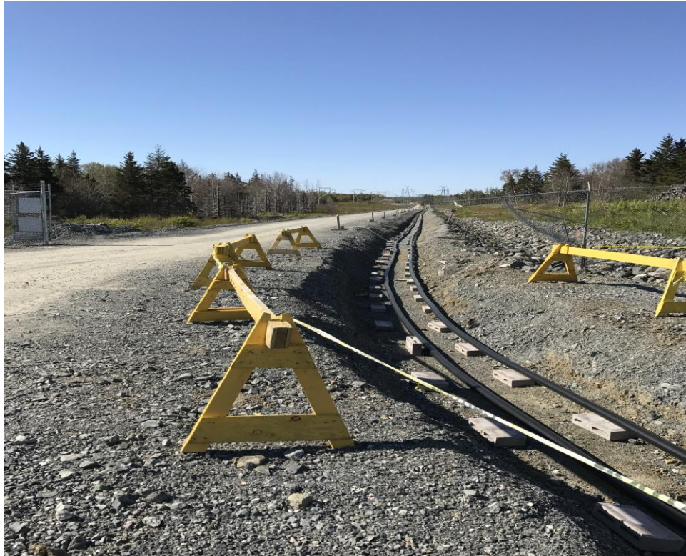
Photo 42: Land cables in position for placement of protective concrete.
