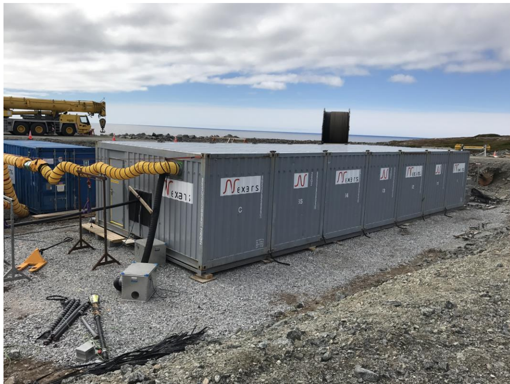
Photo 27: Jointing under controlled conditions of land and subsea Cable 2 (west).
