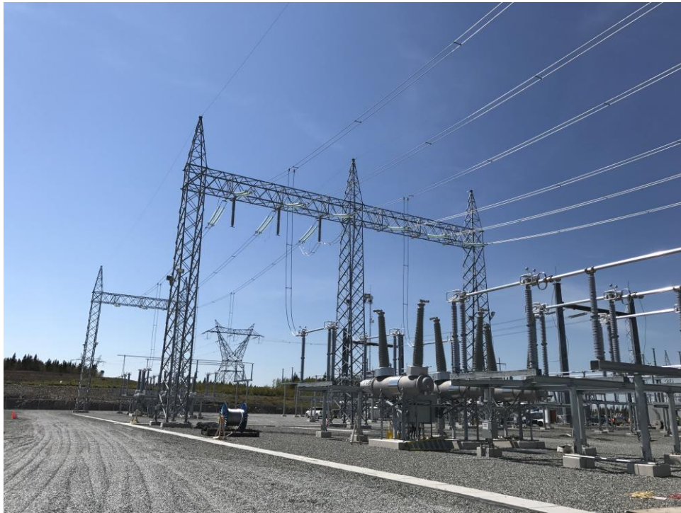
Photos 52: Woodbine - AC Substation work nearing completion.
