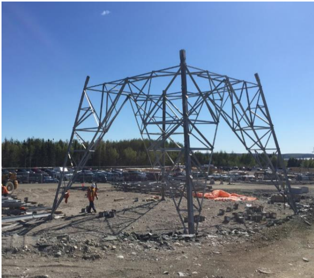
Photos 8/9. Tower assembly outside Bottom Brook.
