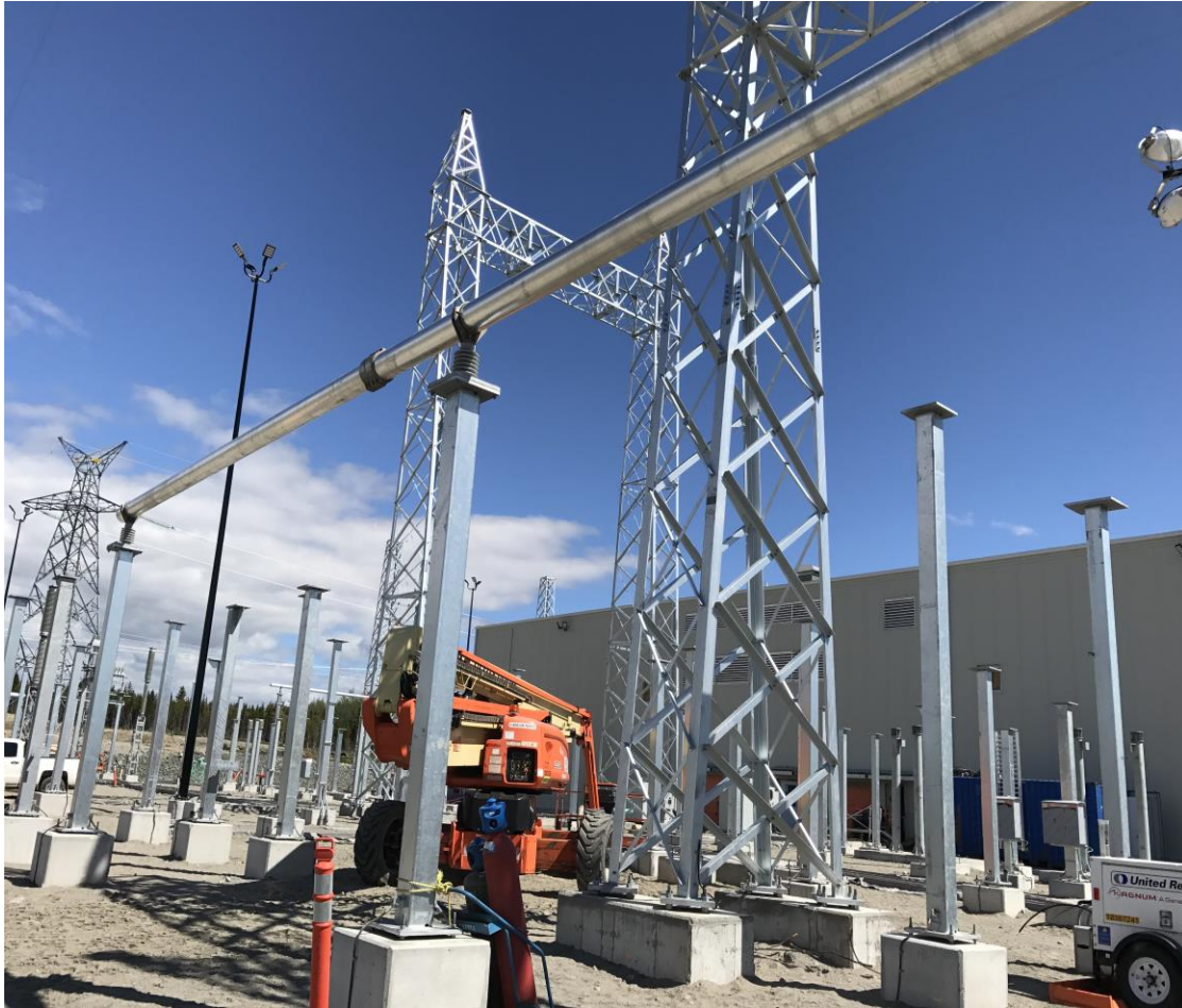
Photo 34: Converter Station building (fully erected) and part of the AC yard.
