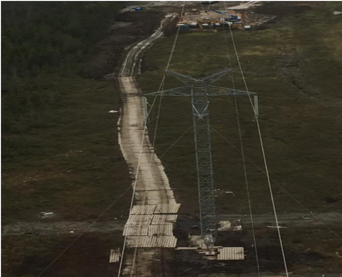
Photo 7. Guyed DC structure / use of access mats due to soil condition.
