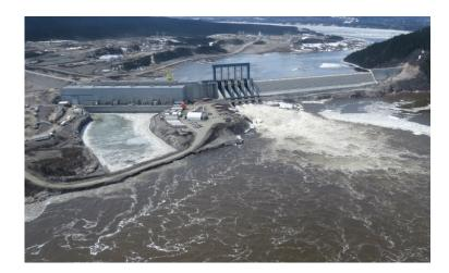
Generating facility – aerial view looking upstream with Powerhouse on the left, Spillway in the centre and North Dam on the right.
