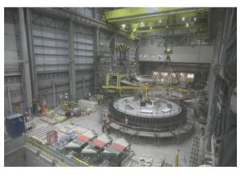
Assembly of turbine and generator parts in the South Service Bay of the Powerhouse
