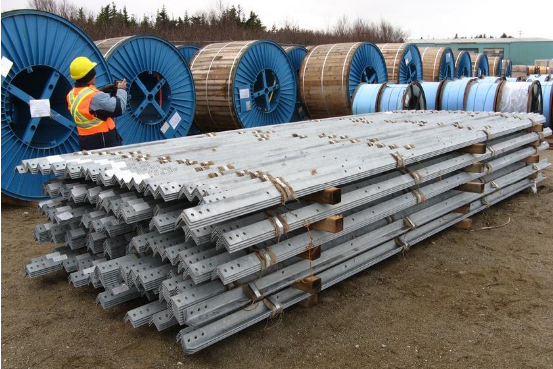
Photo 15: Abengoa materials storage yard - tower steel in foreground; cable drums in background.
