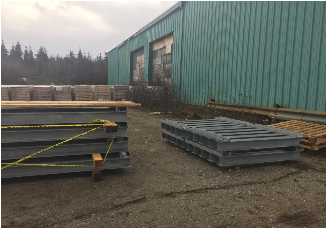
Photo 17: Abengoa materials storage yard – existing building for future preassembly of tower modules.
