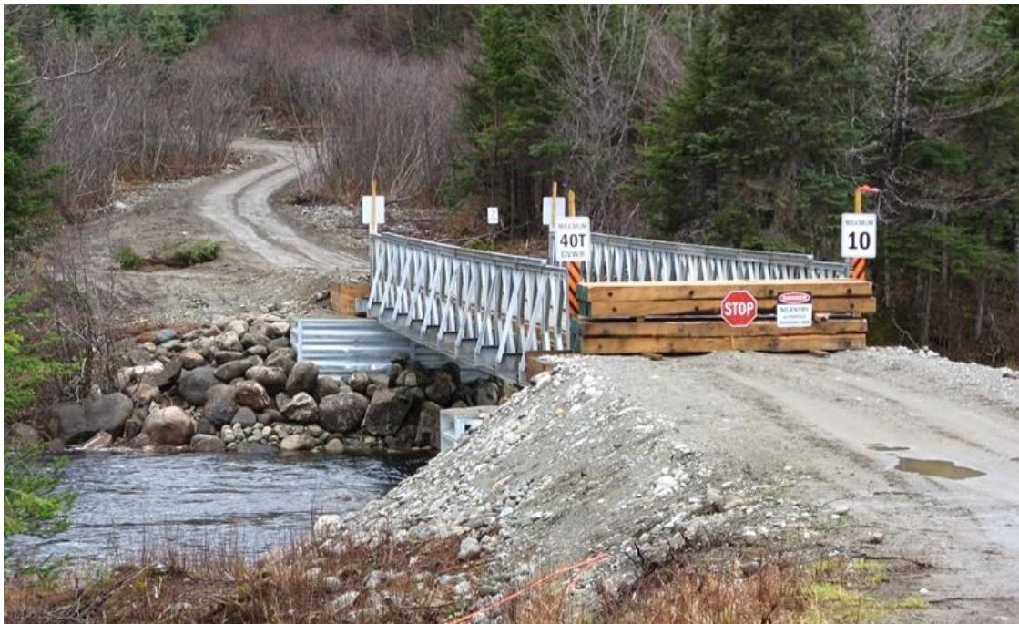
Photo 20: Temporary bridge over Southwest Brook to provide access to HVAC right-of-way.
