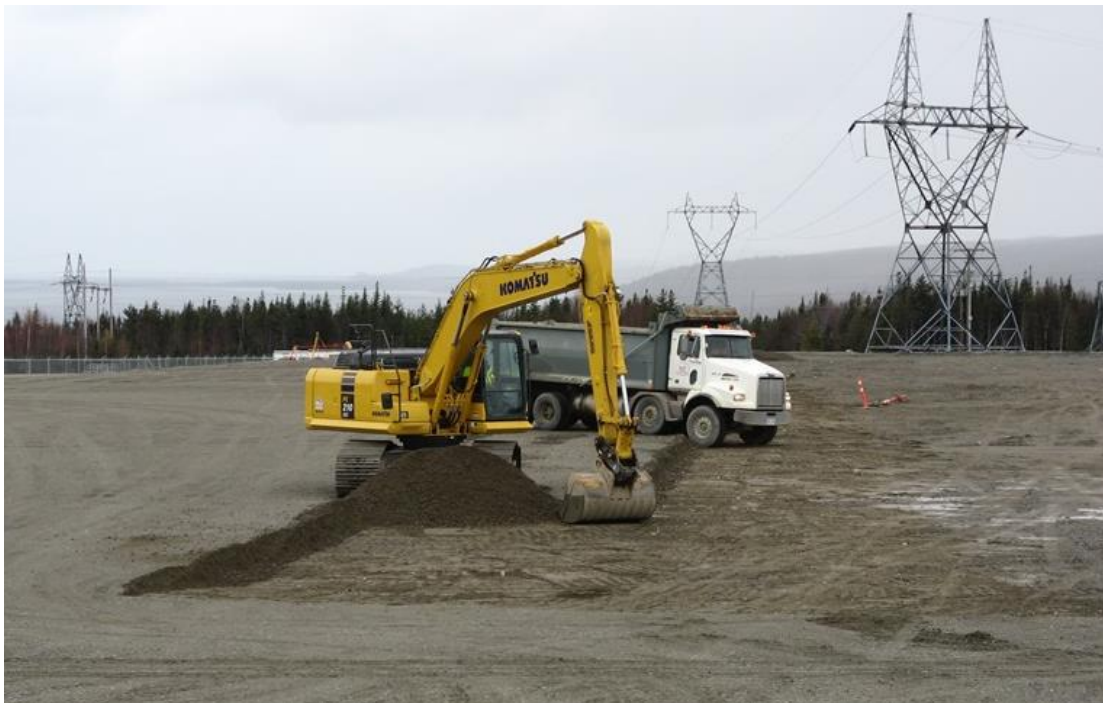
Photo 22: Bottom Brook – temporary stripping of surface running layer in current construction area.
