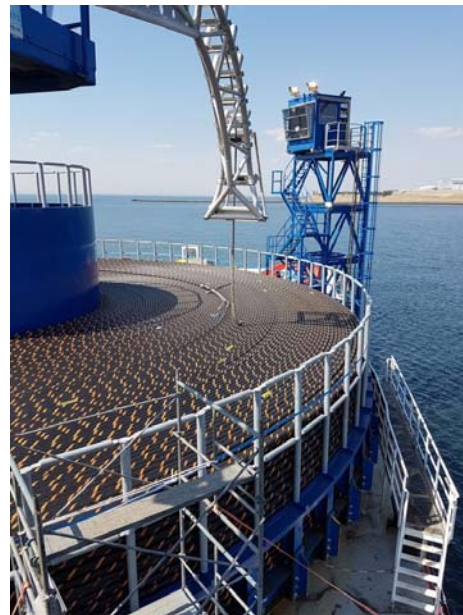
Load out of Cable onto the barge at Futtsu
