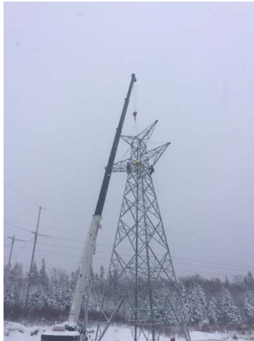
The final tower installed on the NS HVdc line
