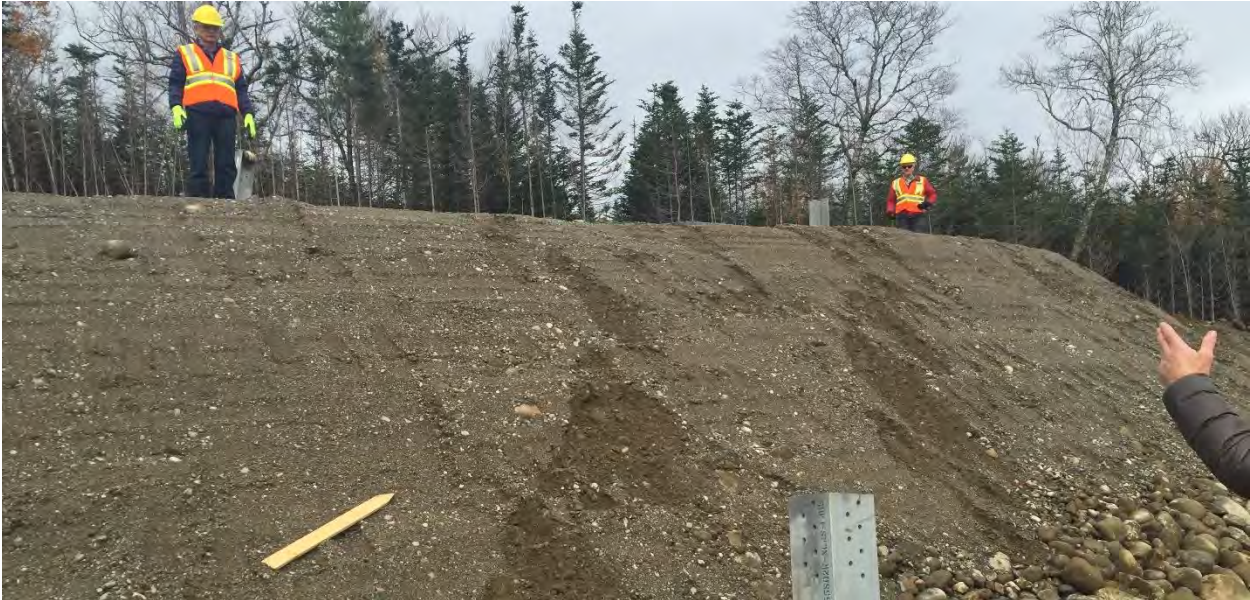
Photos 12 & 13 - HVDC line – steel tower footings installed on sloping ground at site SA7.
