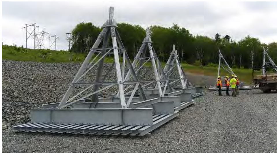
Photo 22 - Assembled type 2 grillages for tower 164 foundation. Rock covered slope in background is typical of permanent erosion protection along roads and ditches.
