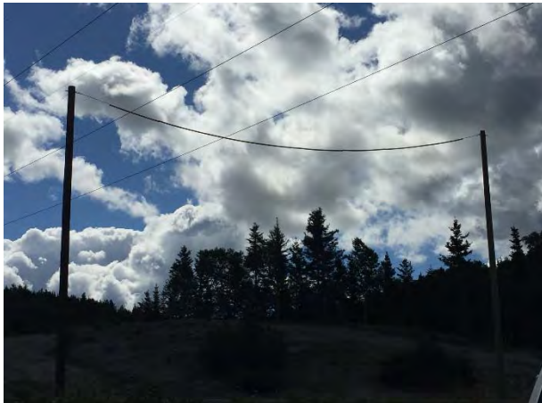
Photo 20 - HVAC line near Granite Canal – Pictures show rider poles used for stringing over roads
