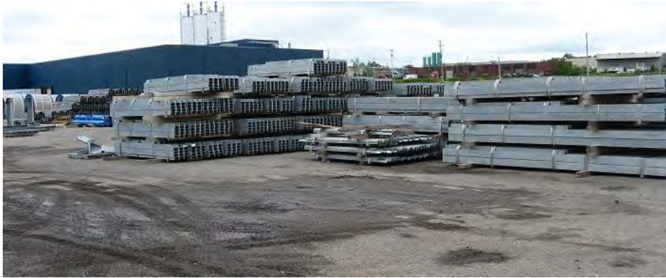
Photo 10 - Grillage and tower steel.
