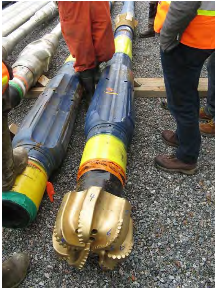
Photo 6 - Drill bit and following drill rod sections. Blue sections contain movable components that are used to steer the drill along its design alignment.
