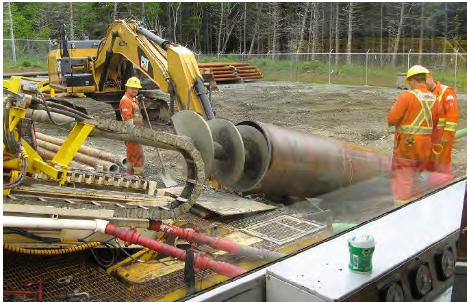
Photo 3 - Auger drill bit used to advance drill hole ahead of casing. Photo is taken from inside of drill operator's control room.
