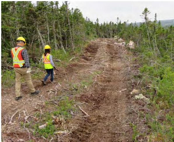
Photo 26 - HVAC line access near Granite Canal – access trail through area of small trees at left, and bog crossing with timber mats at right.
