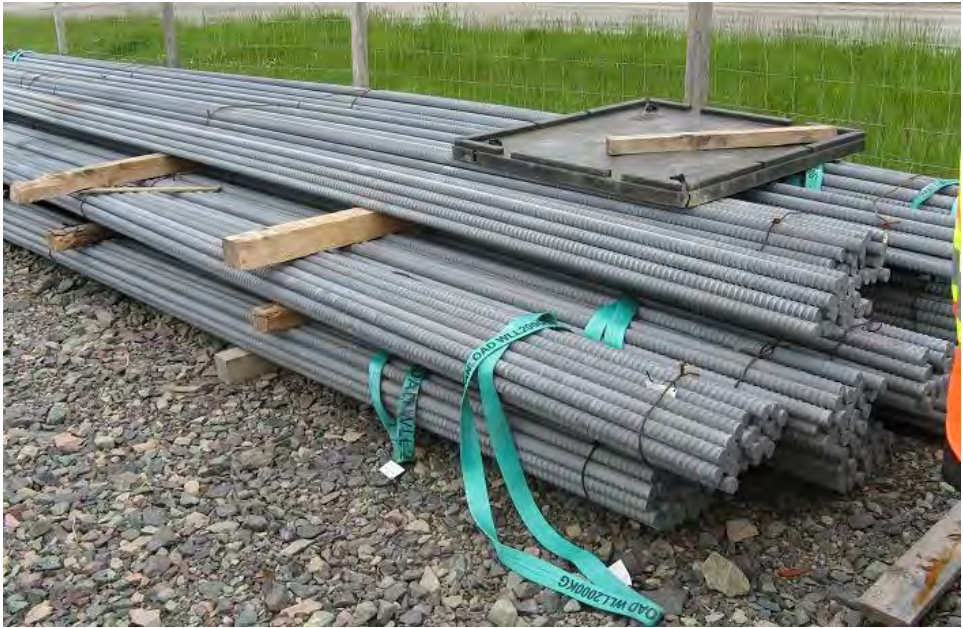
Photo 9 - Threadbar anchors for tower footings.
