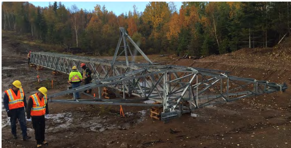
Photos 22, 23 & 24 - Cape Breton HVDC line – assembled guyed tower on ground ready for installation on pedestal foundation at left. Recently installed freestanding tower in centre background.
