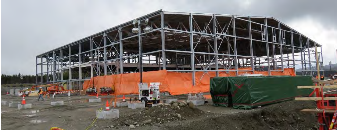
Photo 1 - Bottom Brook –steel frame of converter building.
