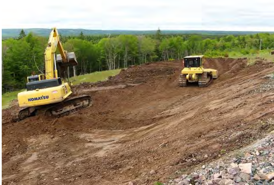
Photo 21 - Foundation preparation for tower 164 (last tower before Woodbine convertor station)
