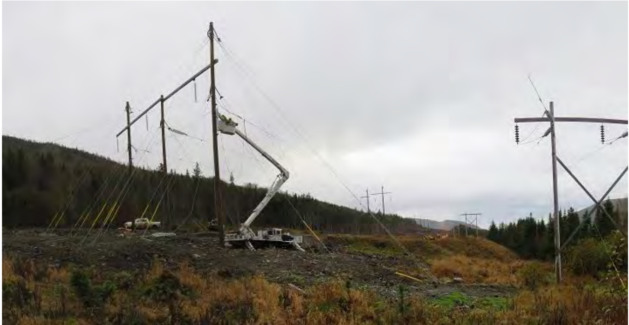
Photo 16 - Westerly view along HVAC line along Burgeo Highway, with Tower 259 at left. Line tensioning of section to Tower 280 is in progress. Existing line at right.
