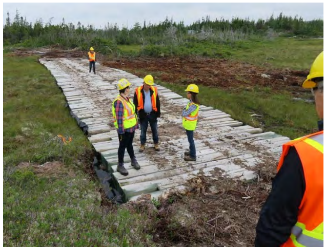
Photo 26 - HVAC line access near Granite Canal – access trail through area of small trees at left, and bog crossing with timber mats at right.
