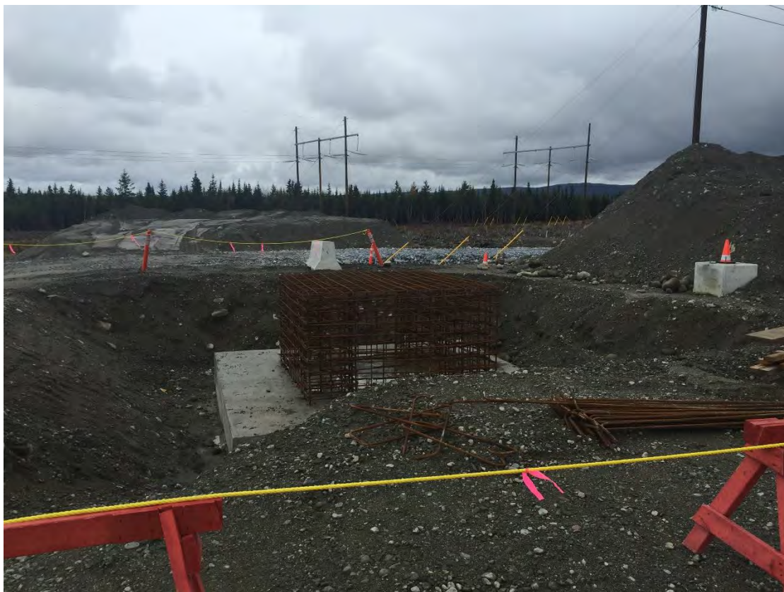
Photo 8 - Bottom Brook – Foundation work for lightning tower.
