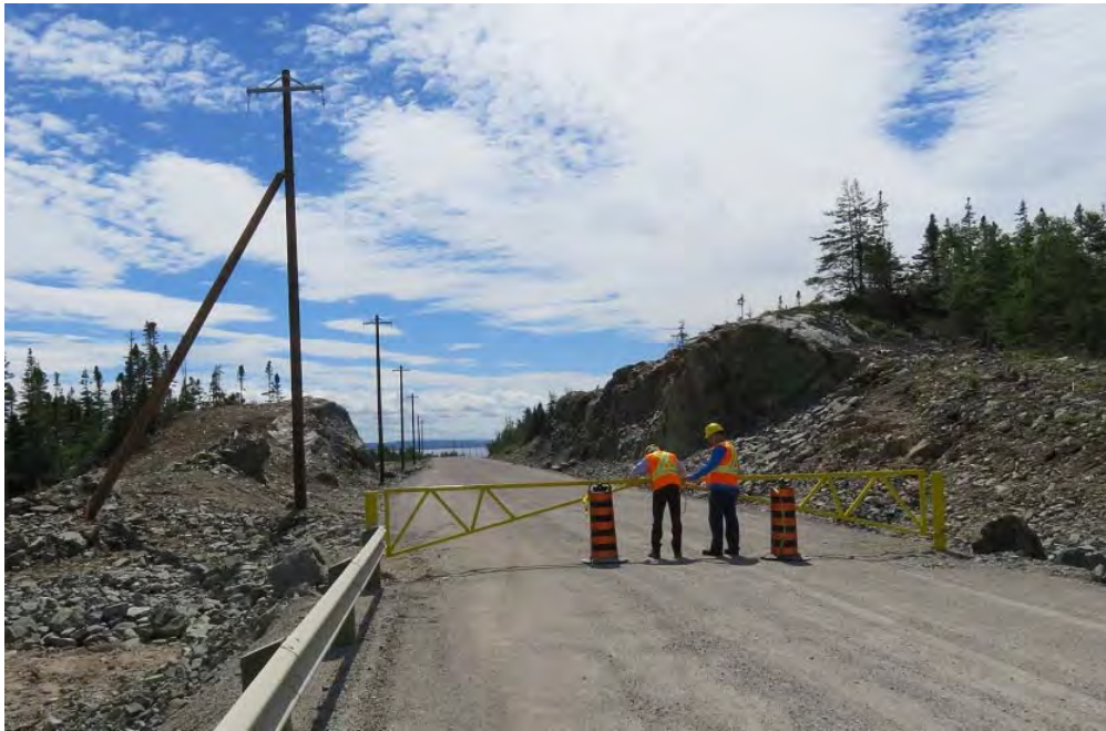
Photo 2 - Indian Head Grounding Site – View along completed site access road towards security gate and Indian Head site. Grounding lines have not yet been strung along this section of road. Showing an angle pole with a stub.
