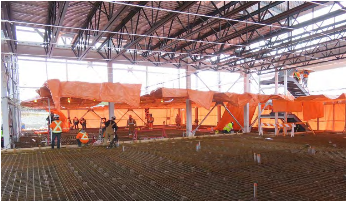
Photo 2 - Bottom Brook – welded wire fabric reinforcement installed in preparation for converter building concrete floor slab placement. Insulated tarps are being installed in background to maintain adequate temperature for concrete curing. Roof trusses and Q deck roof visible at top of photo.
