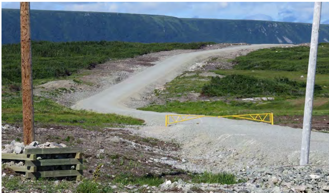
Photo 10 - Cape Ray – view from HDD site looking up completed access road to the transition compound site. The HVDC line between the HDD site and the transition compound will be buried beside the road.
