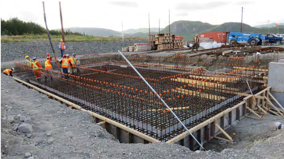
Photo 15 - Bottom Brook – concrete placement in progress for converter transformer foundation. Note safety caps on exposed vertical rebar ends.
