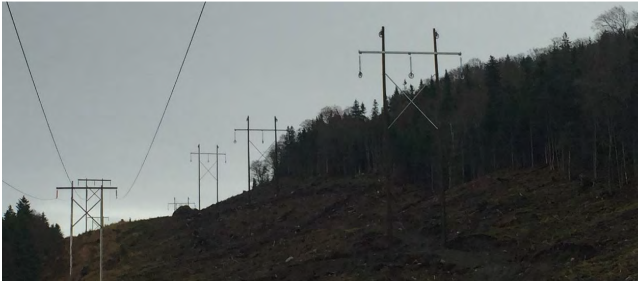
Photo 17 - HVAC – Easterly view looking beyond STR 259. New HVAC line at the right and existing line at left. Structure installation complete and waiting for the stringing.
