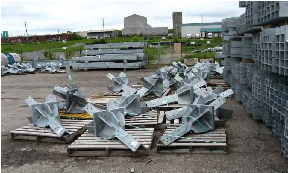
Photo 11 - Grillage footing components.
