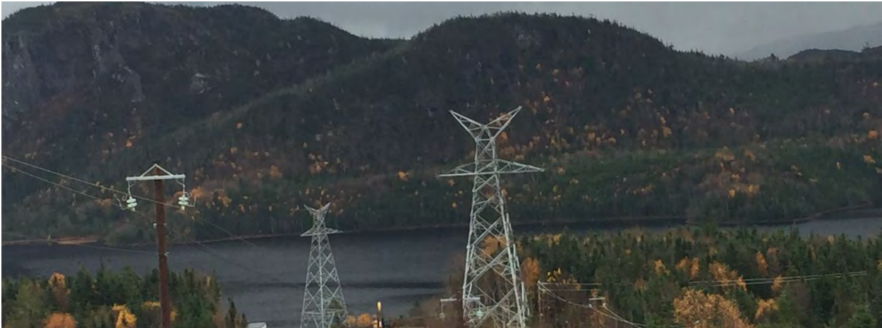
Photo 11 - HVDC line coming to the switchyard.
