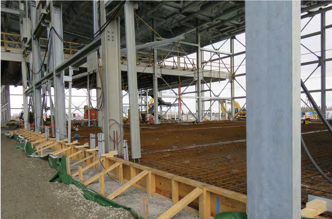
Photo 30 - Woodbine – interior of converter building with concrete floor reinforcement in place in some areas.
