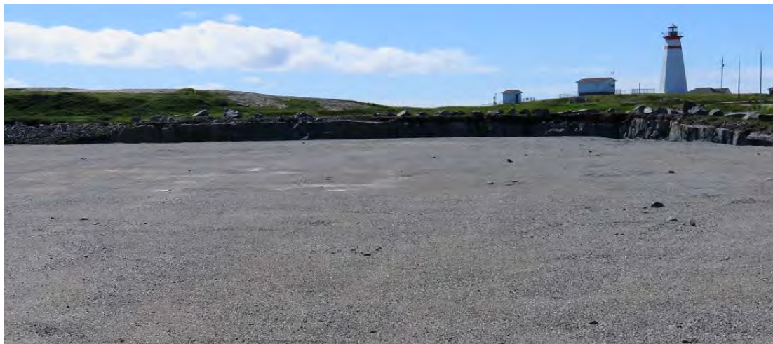
Photo 8 - Cape Ray landfall site – HDD drill pad.
