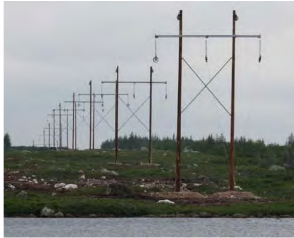
Photo 19 - HVAC line near Granite Canal – completed section of line at left, and poles with pulleys in place, ready for line stringing at right.
