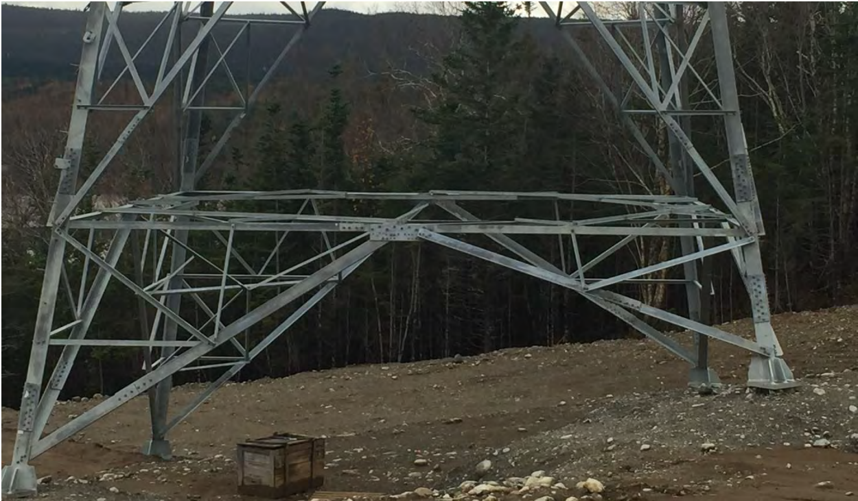
Photo 15 - HVDC – Erected lattice structure tower
