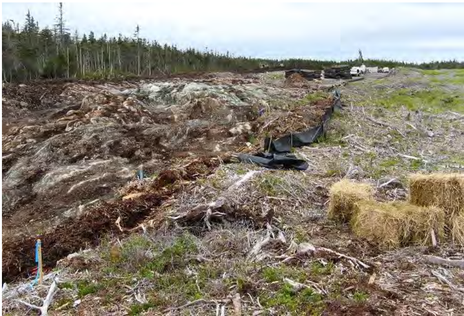
Photo 31 - Access road alignment after stripping of overburden. Silt fences and straw bales are elements of erosion and sediment control. Light grey material in center background is piles of drill cuttings from drilling of blast holes.
