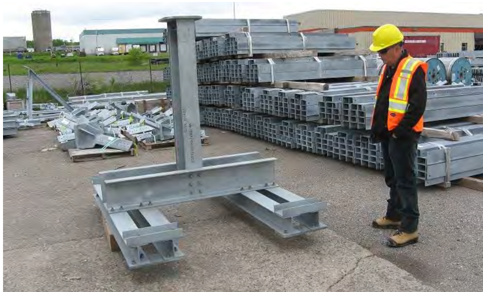
Photo 13 - Type 1 grillage (footing) for rock conditions.
