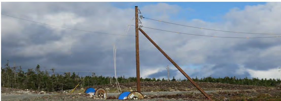
Photo 34 - Big Lorraine grounding site – panorama view inside protective rock berm. Caissons for ground rods are installed below gravel in area behind figures in centre of photo.
