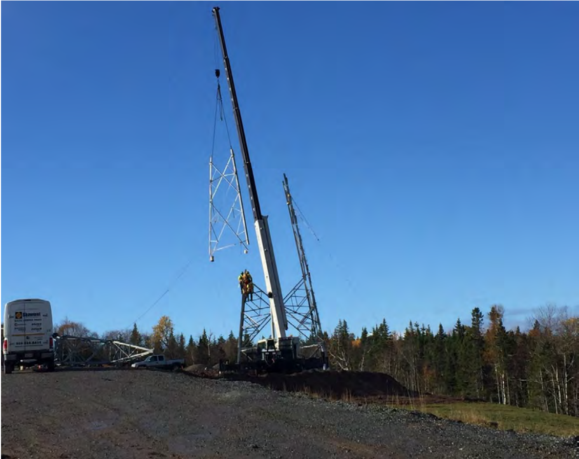
Photo 27 - Cape Breton HVDC line – tower erection in progress adjacent to Woodbine converter station site.
