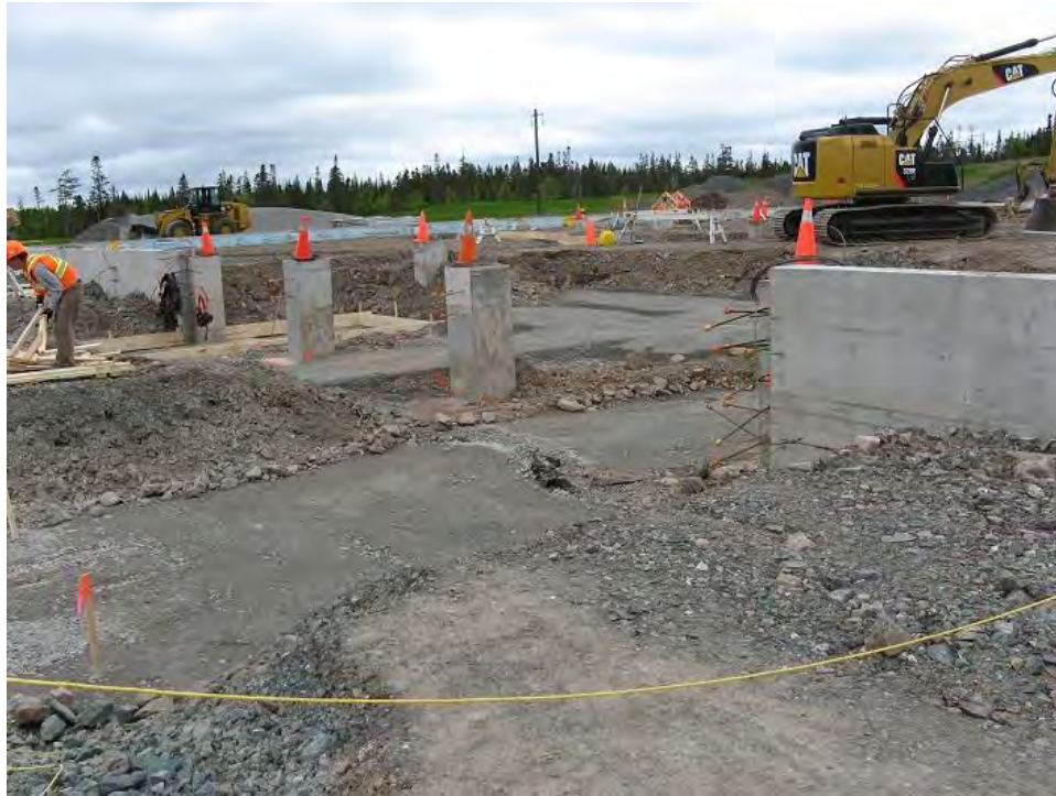
Photo 27 - Converter station foundation.
