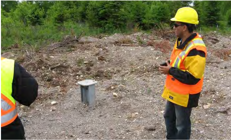
Photo 19 - Pin footing for tower 144.
