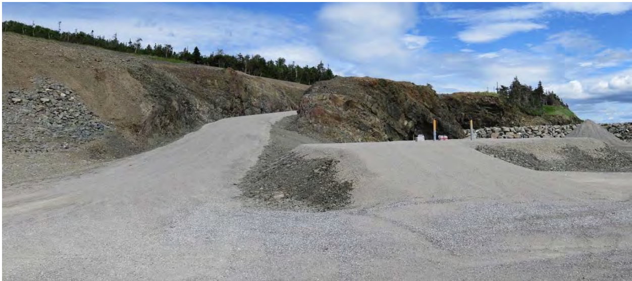
Photo 5 - Indian Head Grounding Site – View looking up access road at left. Overhead lines will terminate at pad at centre right side of photo.
