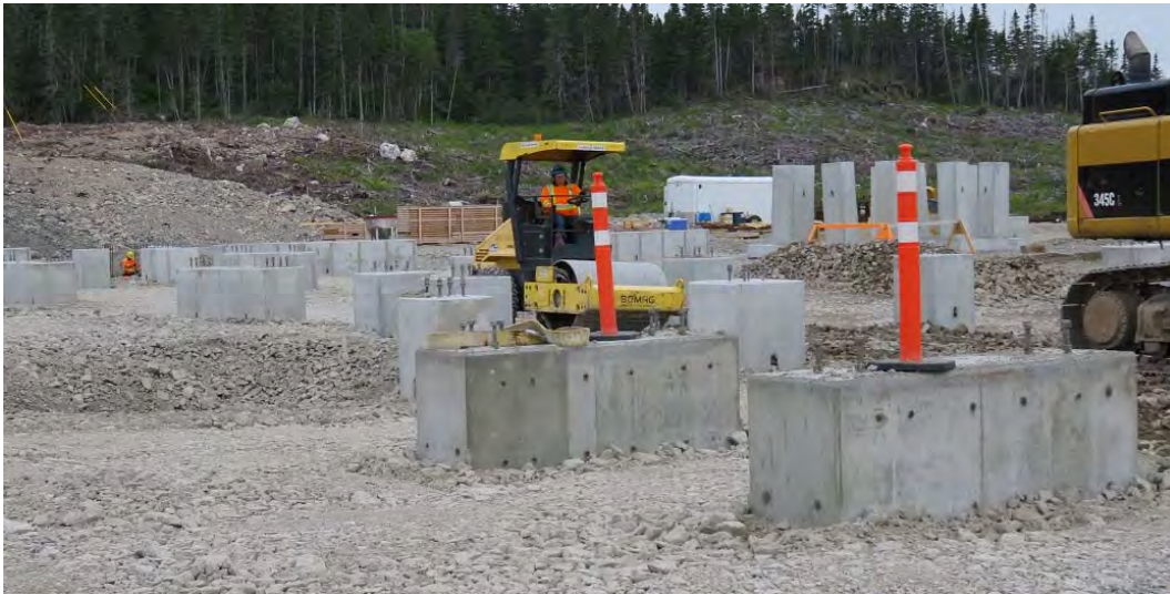
Photo 30 - Granite Canal Switchyard – compacting rockfill around recently-installed precast concrete footings.
