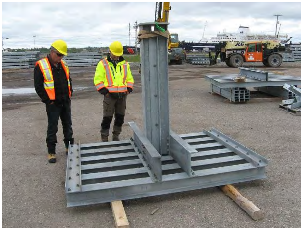
Photo 14 - Type 2 grillage (footing) for soil conditions.
