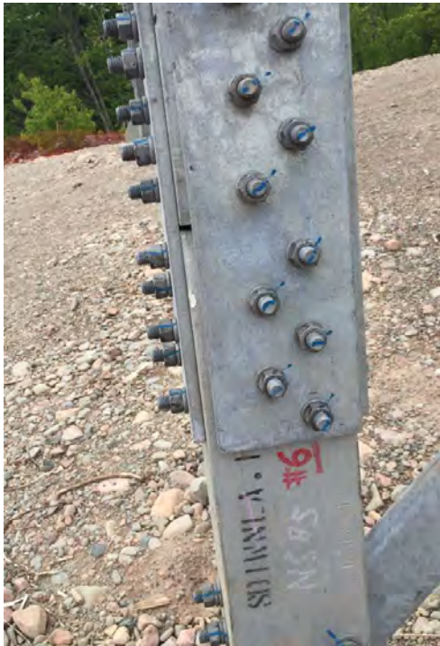
Photo 20 - Marking to confirm the bolt torque
