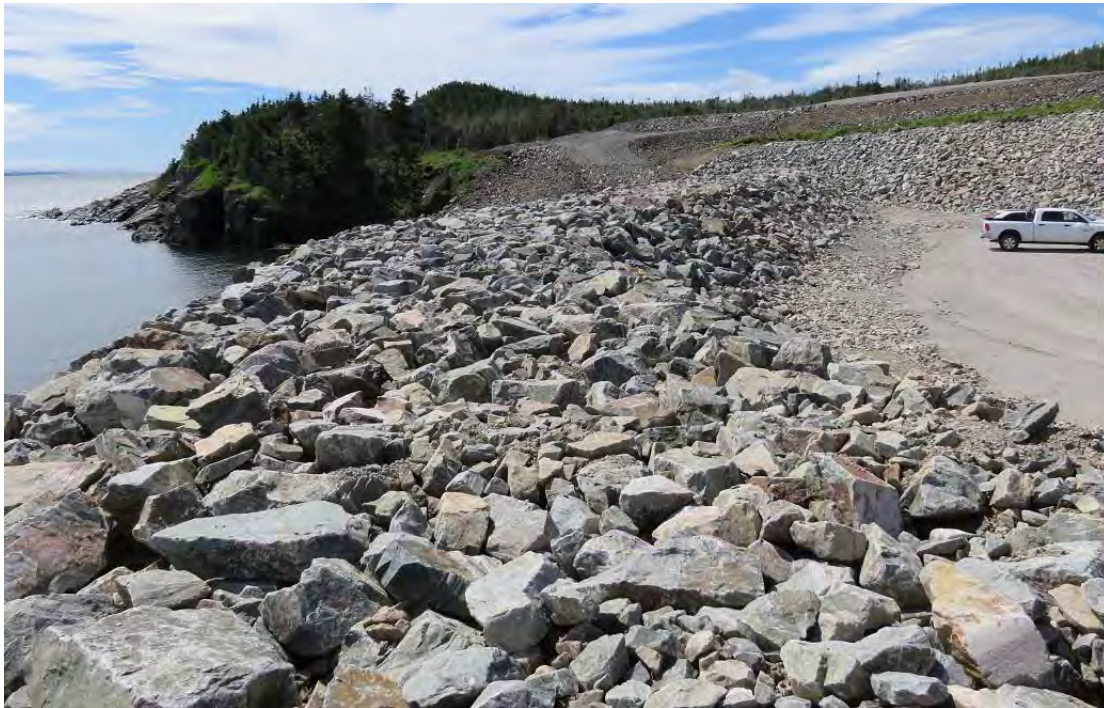
Photo 6 - Indian Head Grounding Site – Protective rock berm constructed in water. Construction access road in background has been decommissioned.
