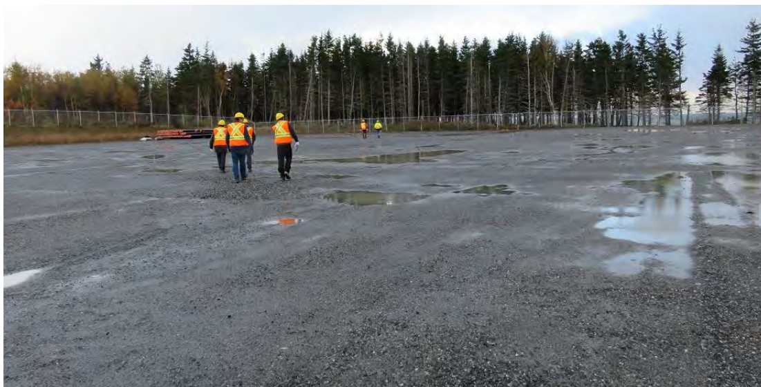
Photo 18 - Point Aconi – landfall site after completion of HDD drilling.
