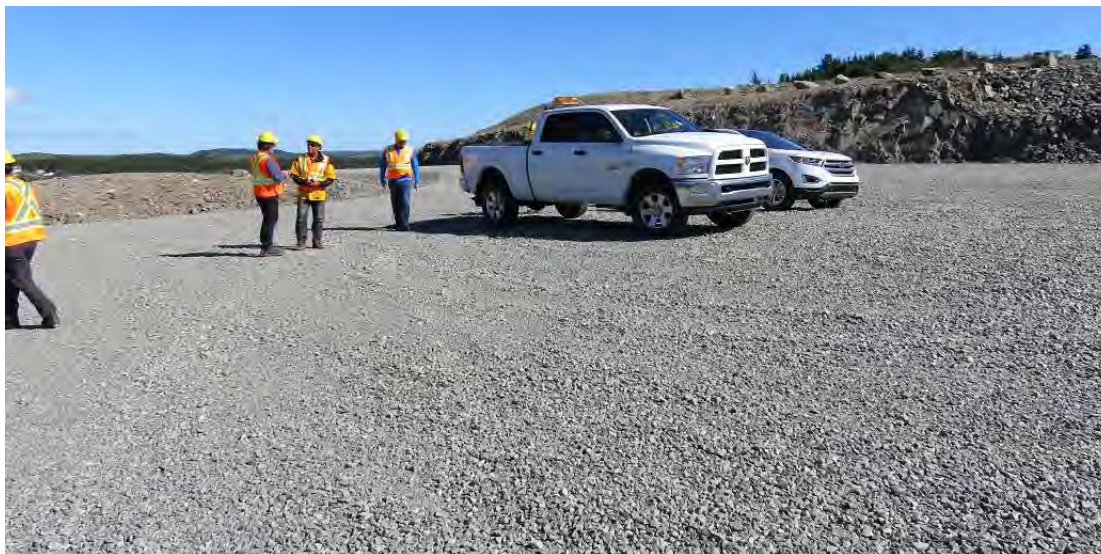
Photo 11 - Cape Ray transition compound – view looking across compound site towards access road.
