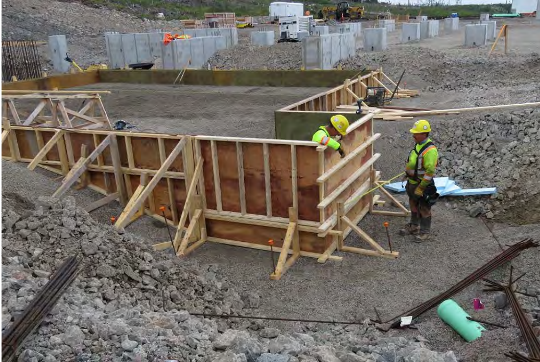
Photo 31 - Granite Canal Switchyard – Construction of formwork for concrete foundation for shunt reactor equipment.
