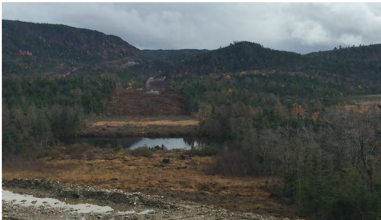
Photo 10 - HVDC line – Right of way clearing
