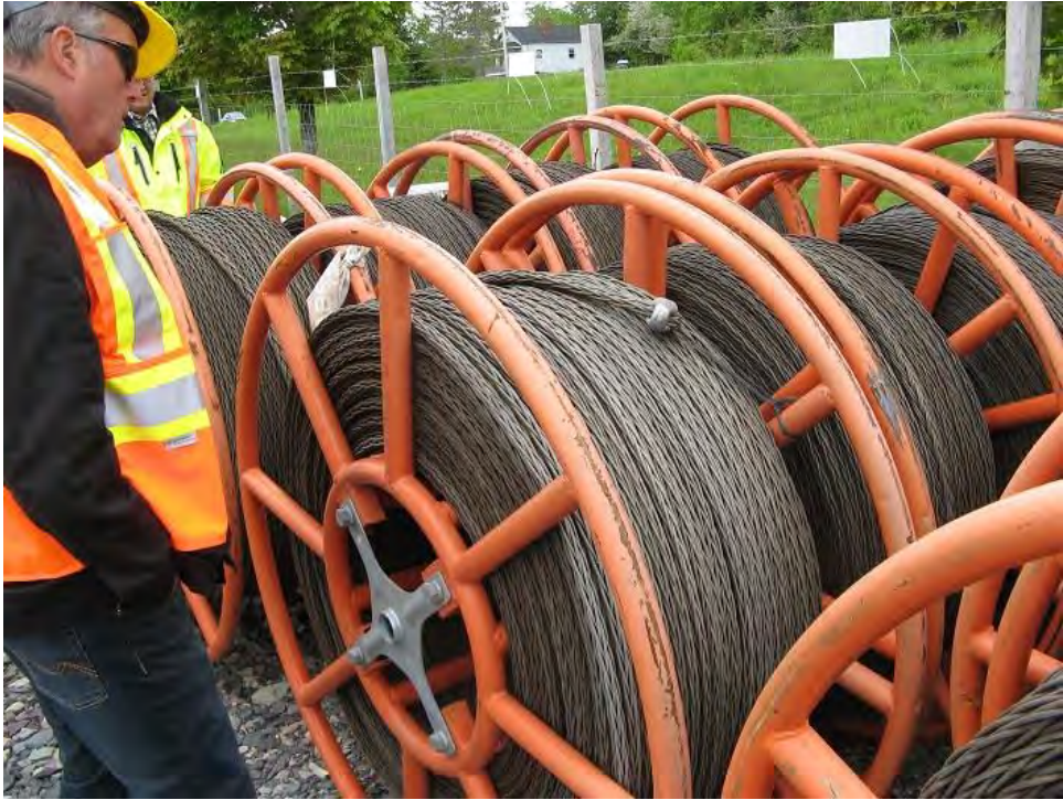
Photo 8 - Guy wire for towers.
