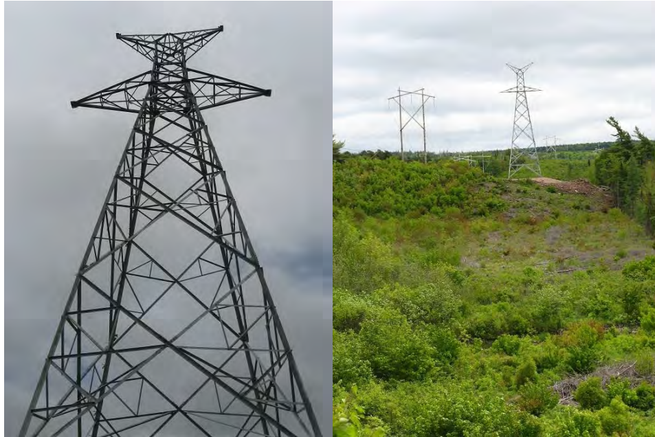
Photo 17 - Tower 151 (left) and adjacent tower (right).
