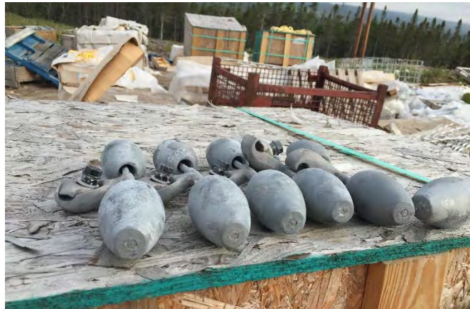
Photo 24 - HVAC line near Granite Canal – Picture on the left shows some of the materials (grounding rods and armor rods) and the picture on the right shows the vibration dampers.
