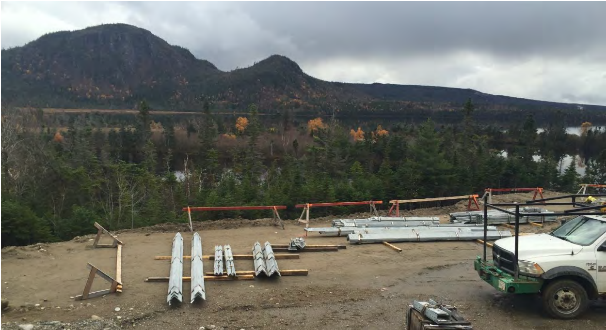
Photo 14 - HVDC – Structural members ready for tower assembly
