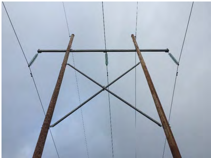
Photo 22 - HVAC line near Granite Canal – typical wood pole tangent structure (to the right) and dead-end structure to the left
