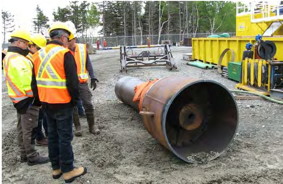
Photo 4 - Casing hammer used to drive 42-inch casing.
