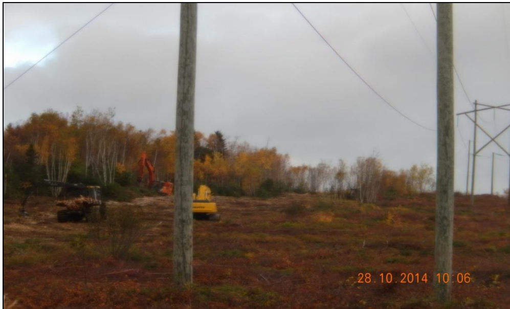
Clearing & widening of the existing transmission ROW
