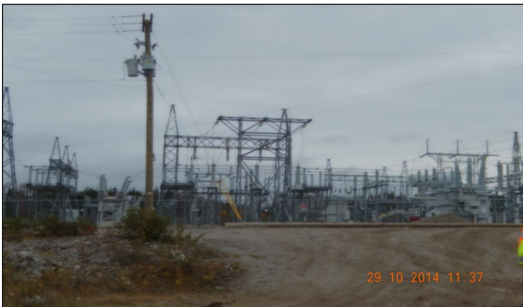
Existing Bottom Brook Terminal Station
