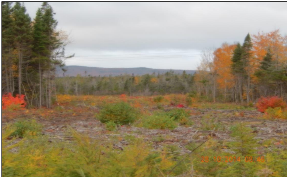
Site clearing for HDD and Transition Compound at Point Aconi
