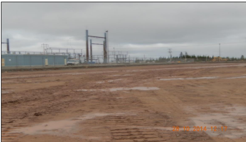
Site preparation for Woodbine Station expansion and converter Station
