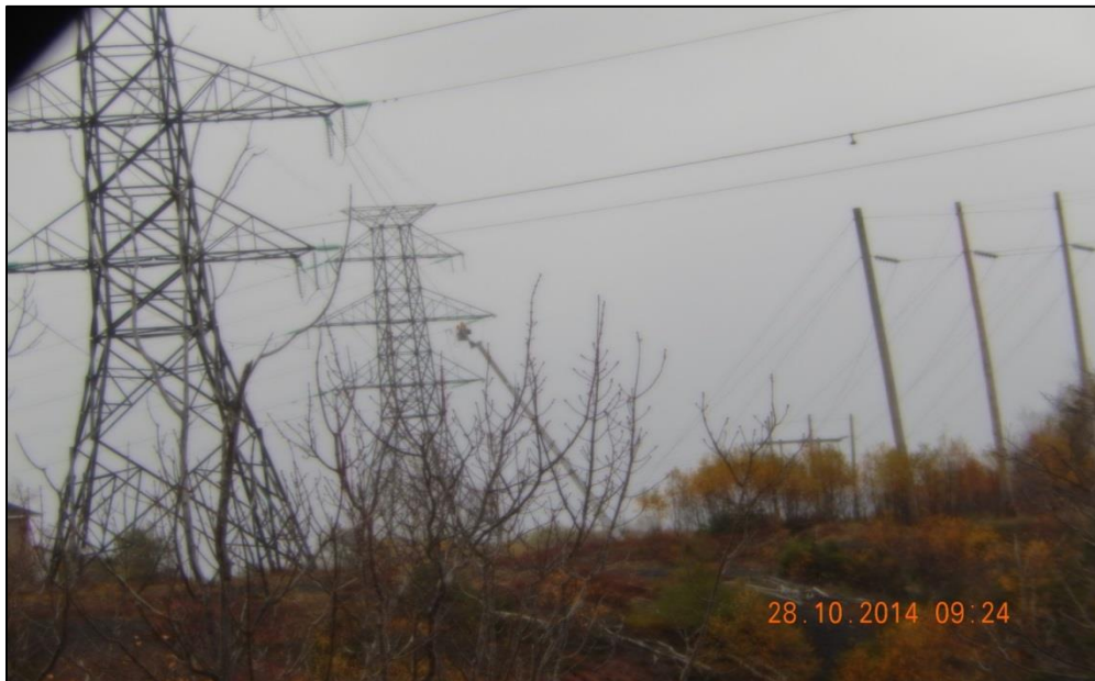
Transmission line being transferred to steel tower
