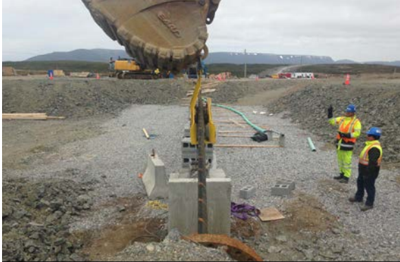
Submarine cable pulled into shore in Cape Ray
