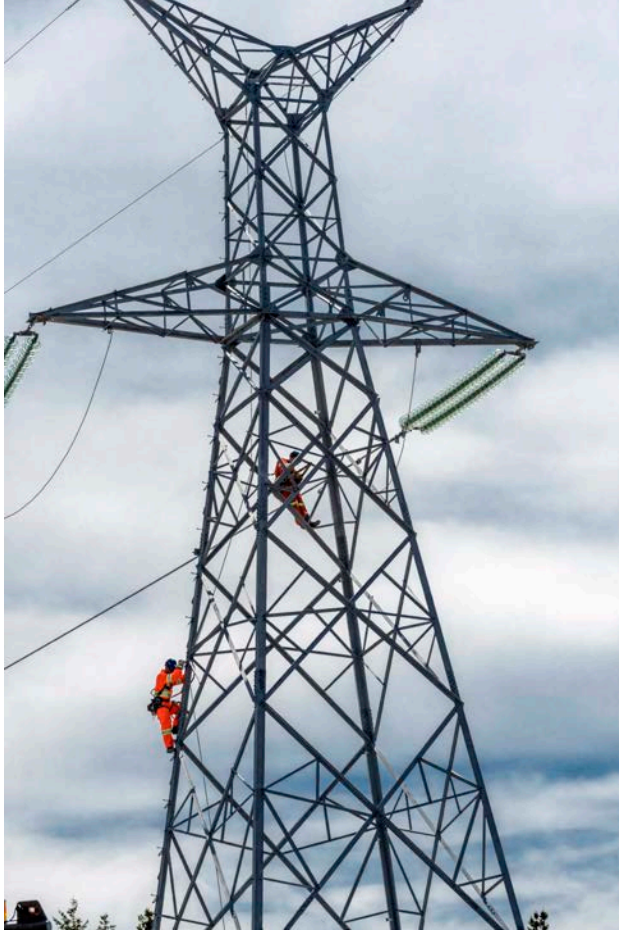
Transmission stringing in Nova Scotia
