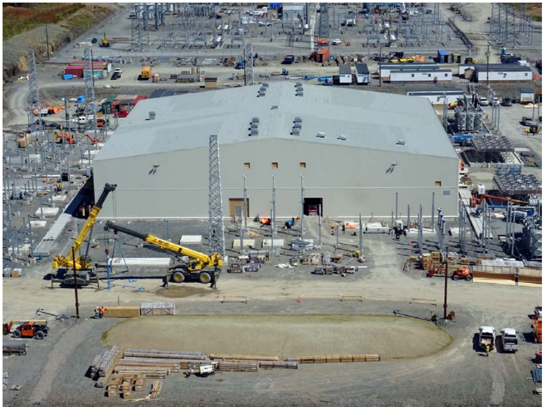
Woodbine Converter Building
