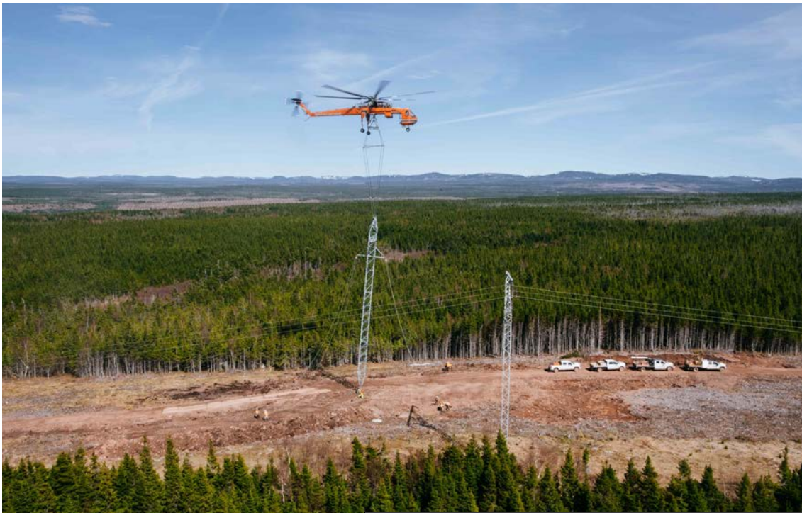
SkyCrane transmission tower lift
