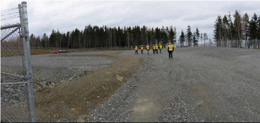
Photo 13: Point Aconi completed landfall site enclosed by security fence. HVDC cables are buried under low berm at left.
