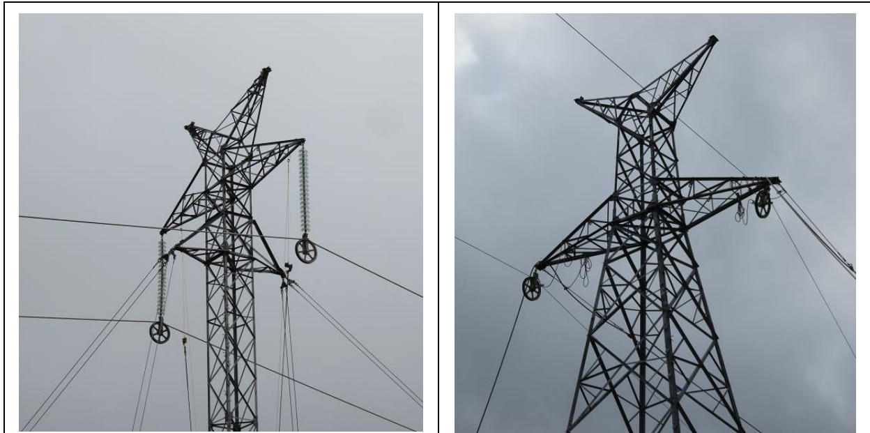
Photo 5: Line stringing in progress on guyed and freestanding HVDC towers.
