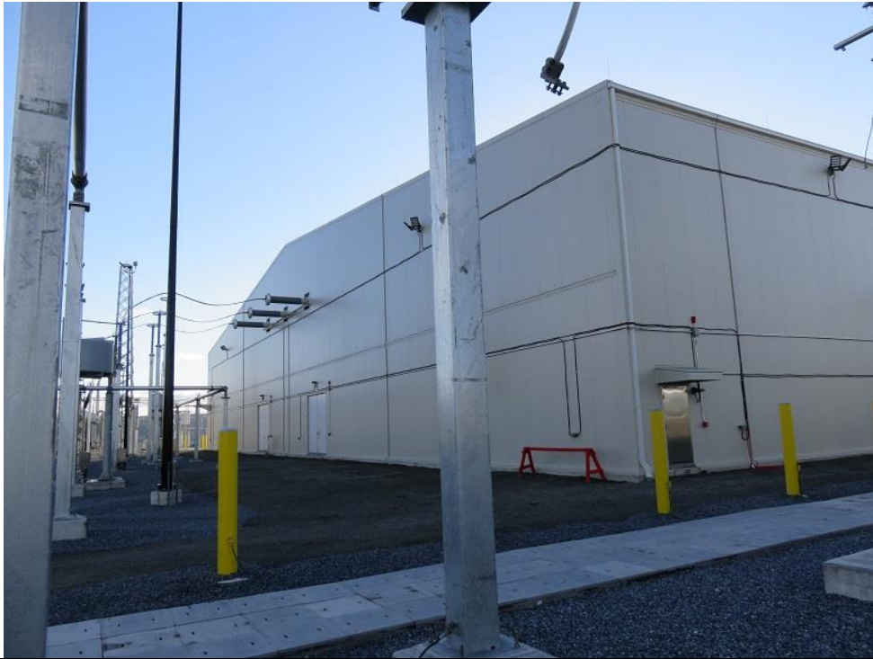
Photo 7: Bottom Brook converter building.
