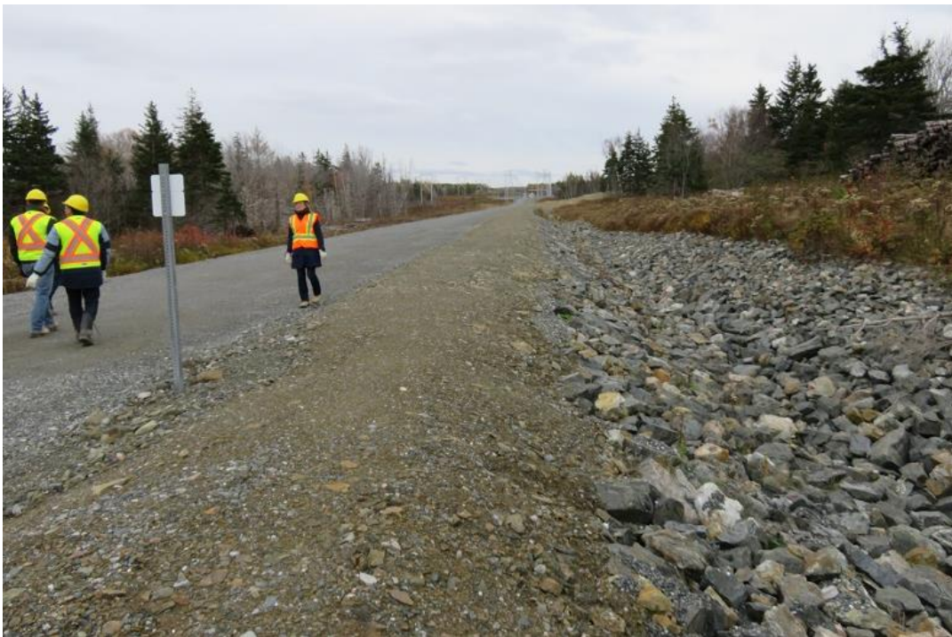
Photo 14: Point Aconi view from landfall site along road to transition compound. Low berm along right side of road covers the buried HVDC land cables, with riprap-lined drainage ditch to the right.
