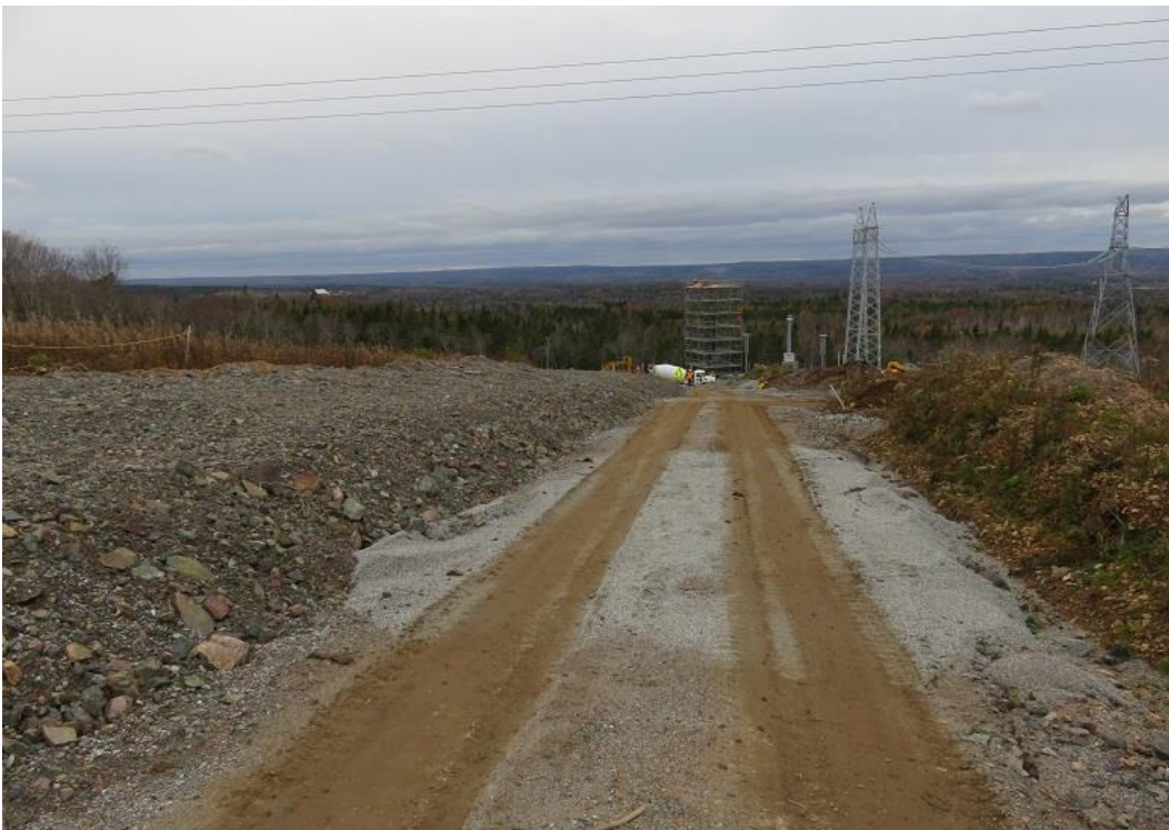
Photo 19: View from Woodbine along construction access road from Woodbine switchyard to HVDC transition structure. Underground HVDC land cables are buried by berm along left side of road.
