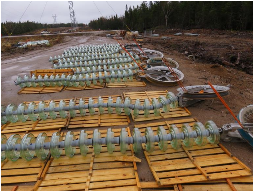
Photo 4: Insulators with attached pulley systems ready for installation along HVDC line.
