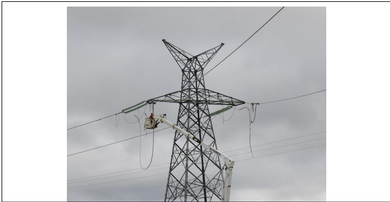
Photo 6: Powerline Technician completing insulator installation on HVDC tower.
