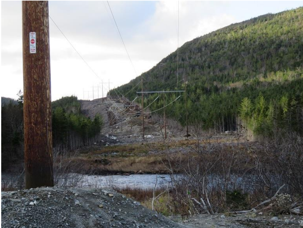
Photo 1: HVAC line at crossing of Southwest Brook along Burgeo Highway, with three-pole angle structures in foreground and two-pole structures in background.
