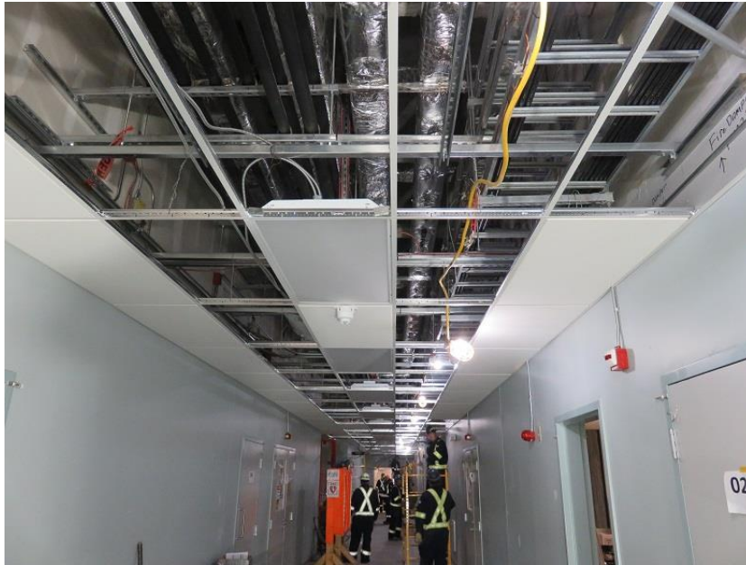
Photo 22: Cable installation works nearing completion inside Woodbine converter building.
