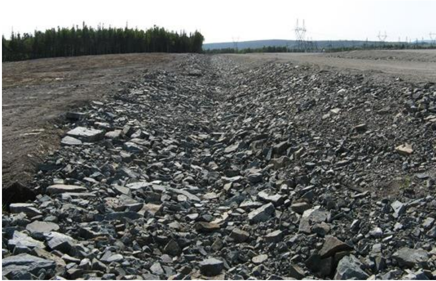
Photo 18 – Bottom Brook – Typical perimeter ditch lined with riprap.
