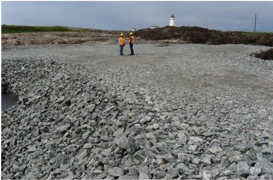
Photo 11 – Cape Ray – HDD site.
