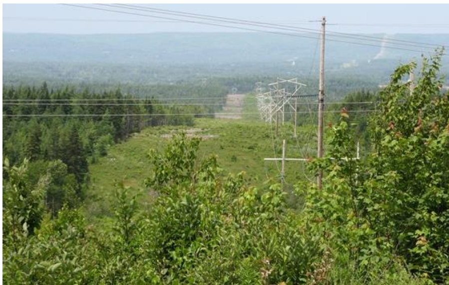
Photo 4 – Cleared right of way adjacent to existing 230 kV line near Woodbine substation.
