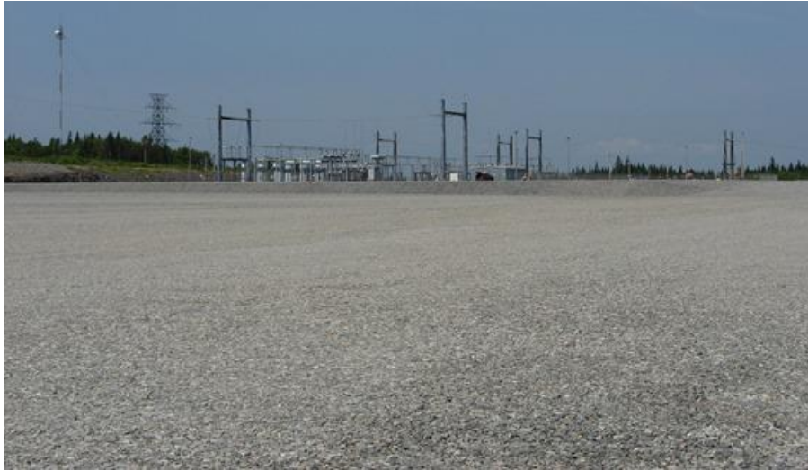
Photo 6 – Woodbine – Prepared site for converter station adjacent to existing substation.
