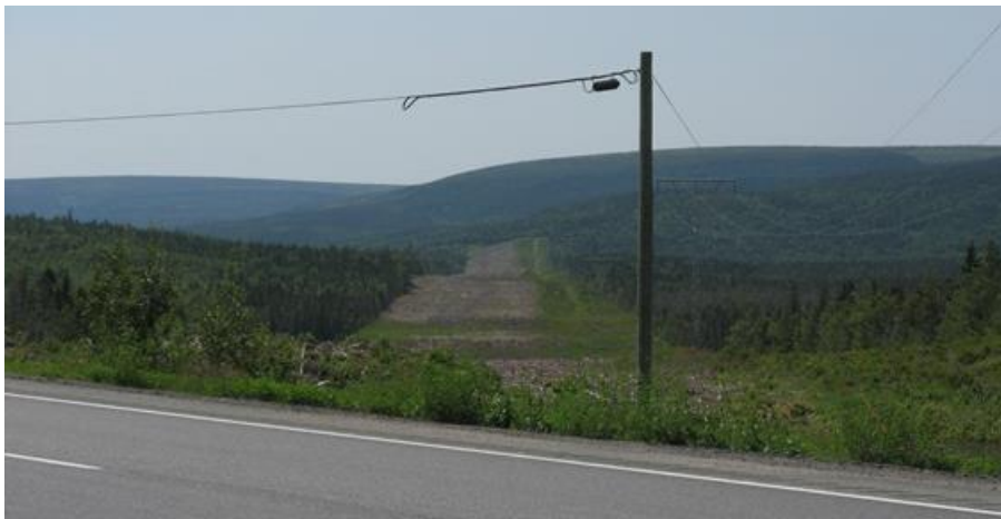
Photo 16 – Typical section of cleared right-of-way for 200 kV HVDC line near Cape Ray.
