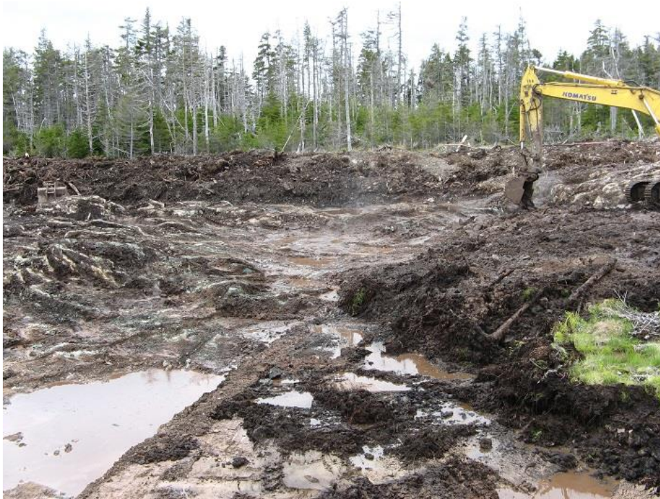
Photo 30 - Overburden stripping of access road alignment in progress.
