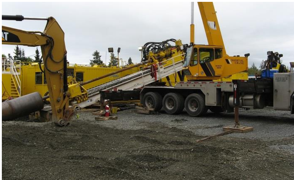
Photo 1 – HDD drill rig installing surface casing at 16 degrees below horizontal.
