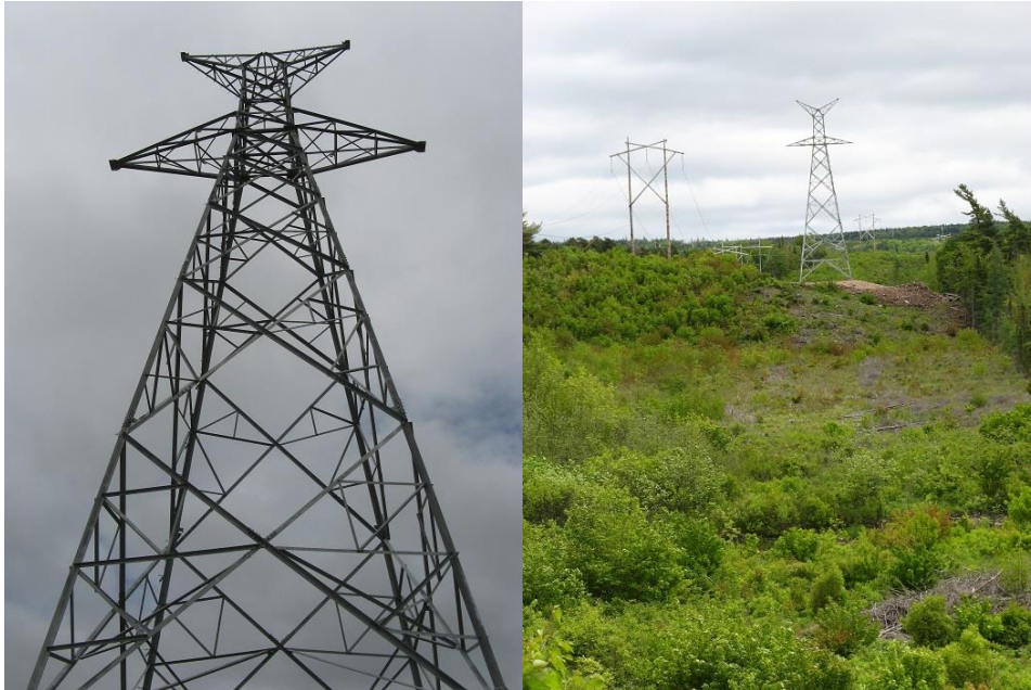
Photo 17 - Tower 151 (left) and adjacent tower (right).
