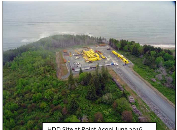
HDD Site at Point Aconi June 2016
