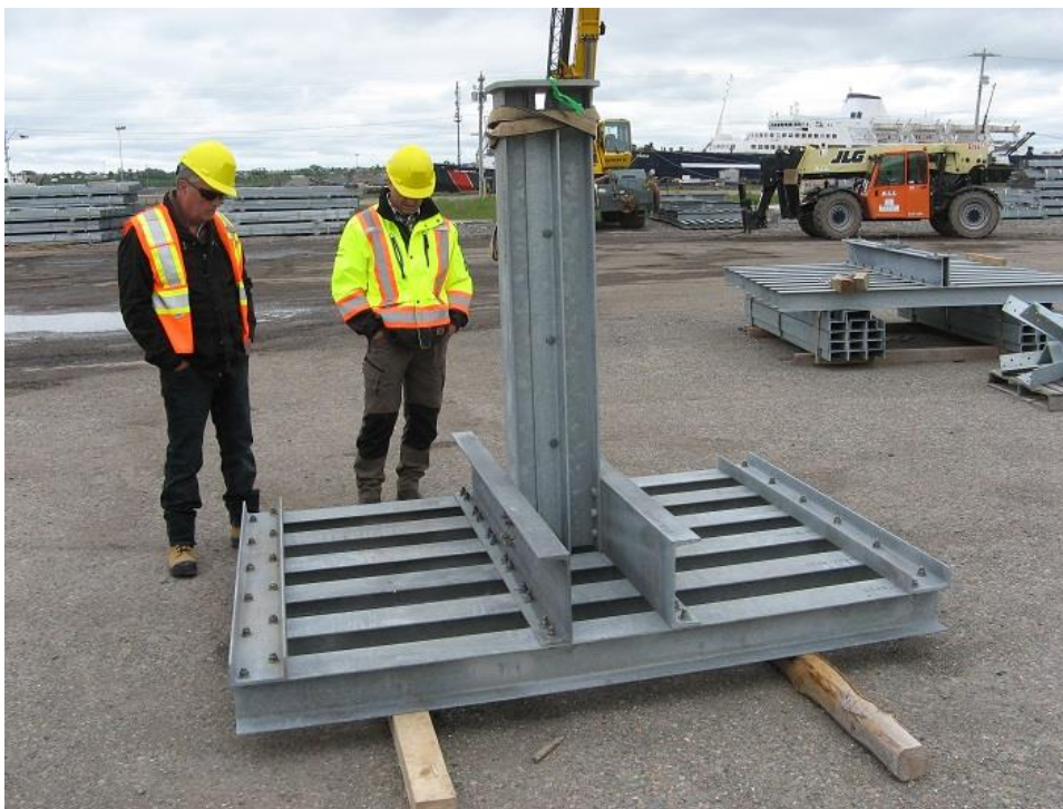
Photo 14 - Type 2 grillage (footing) for soil conditions.
