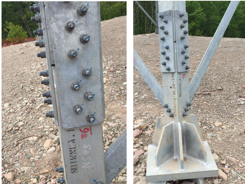
Photo 20 - Marking to confirm the bolt torque
