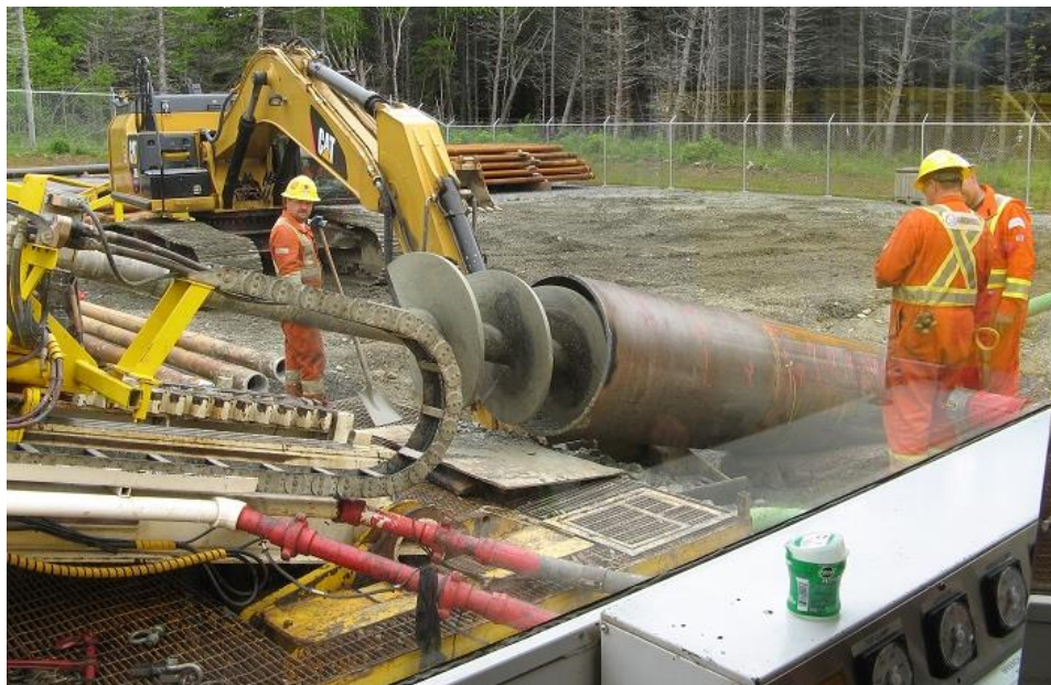
Photo 3 - Auger drill bit used to advance drill hole ahead of casing. Photo is taken from inside of drill operator's control room.
