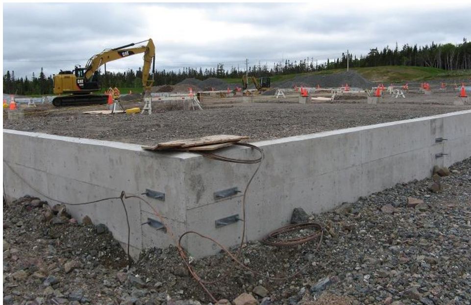
Photo 26 - Converter station concrete foundation ready for the building steel structure erection.
