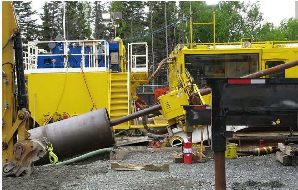
Photo 2 - Large 42-inch diameter pipe is a steel casing. Smaller pipe inside casing is the drill rod which connects to a 36-inch diameter auger bit being used to drill the pilot hole. Drill operator is located in glass booth at right side behind drill rig.
