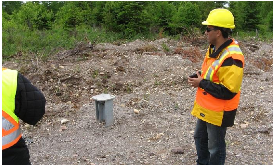
Photo 19 - Pin footing for tower 144.
