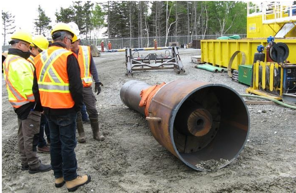
Photo 4 - Casing hammer used to drive 42-inch casing.
