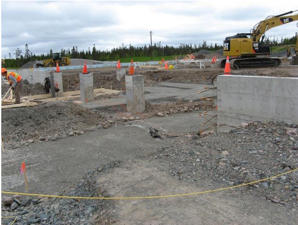
Photo 27 - Converter station foundation.
