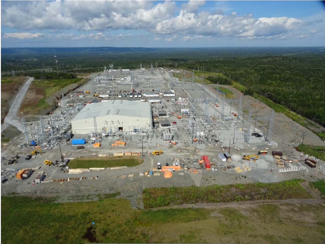
Converter Substation at Woodbine, NS
