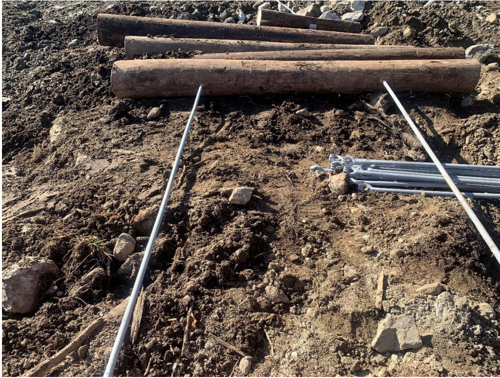
Photo 6: Log anchor for anchor installation
