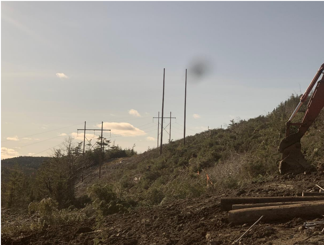
Photo 5: New structure being installed
