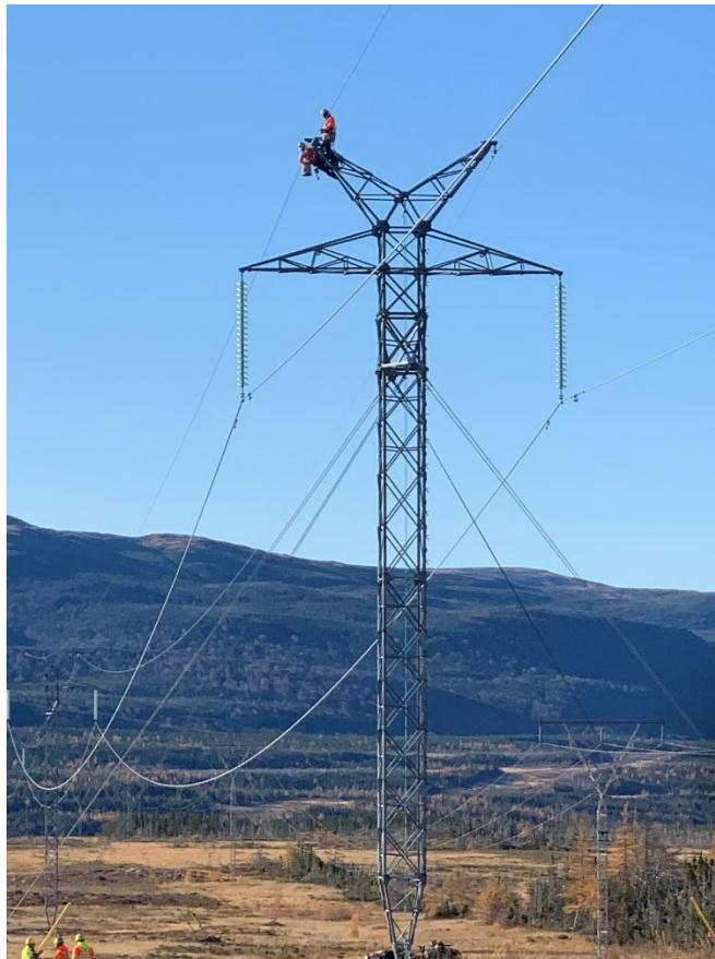
Photo 4: Crew is replacing the damaged shield wire / OPGW clamp at STR 290
