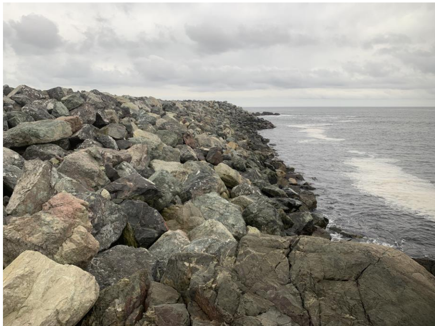
Photo 5: Grounding site – outer side of protective berm in good condition.
