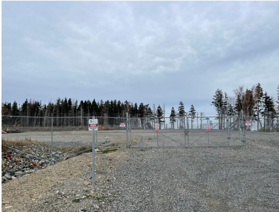
Photo 1: Landfall HDD cables site.
