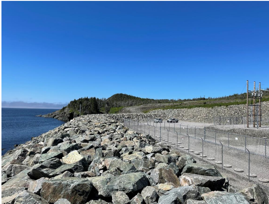
Photo 9: Indian Head grounding site with the protective berm in good condition
