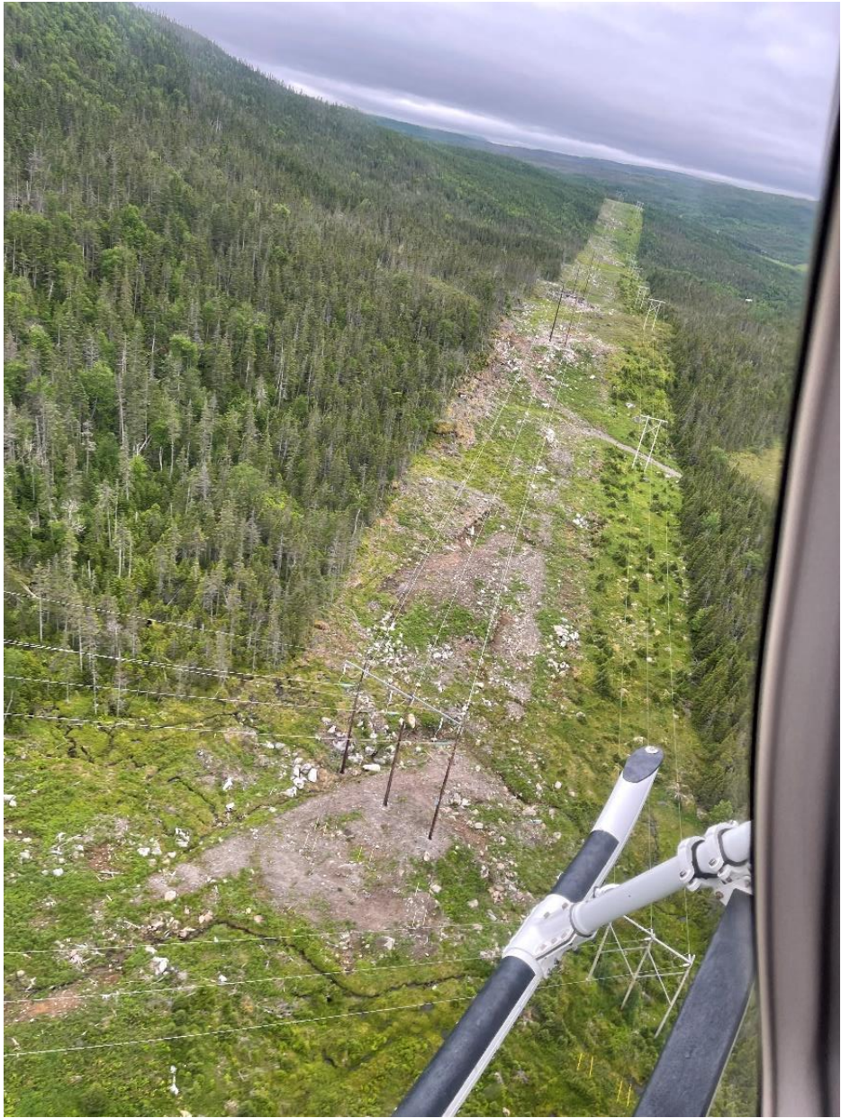
Photo 5: Aerial photo of the AC transmission line
