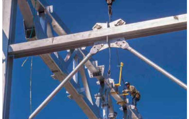
Steel installation progresses for the converter station at Woodbine site.
