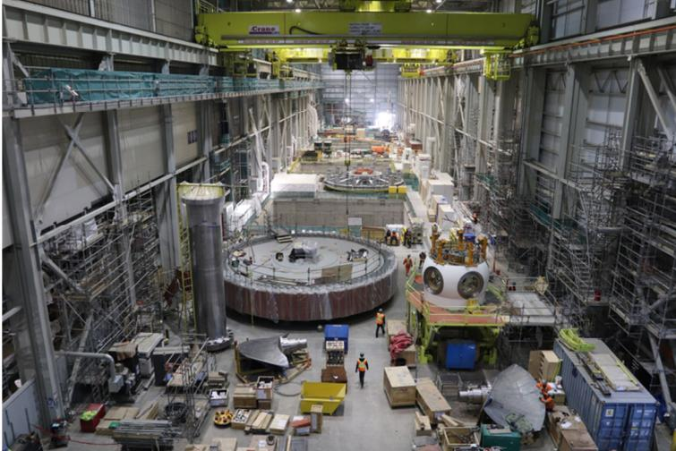
Assembly of turbine and generator parts in the South Service Bay of the Powerhouse
