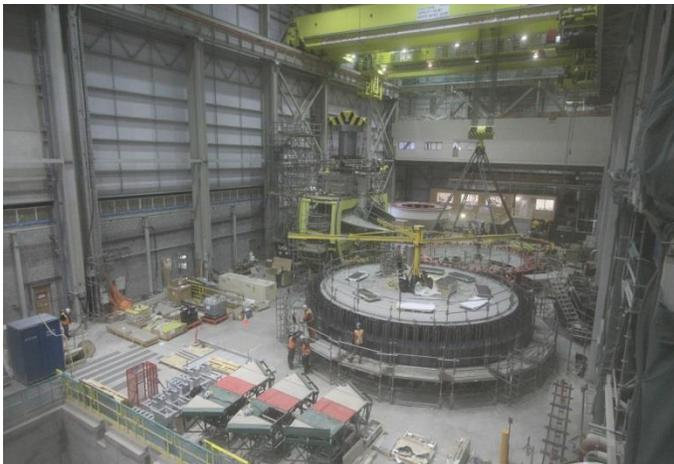
Assembly of turbine and generator parts in the South Service Bay of the Powerhouse
