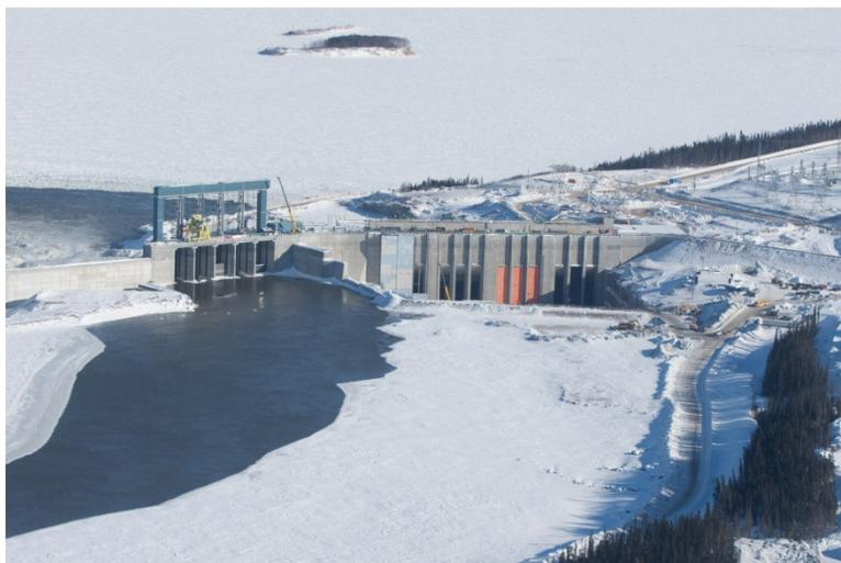
Upstream view of the Spillway (left) and Intake (right)
