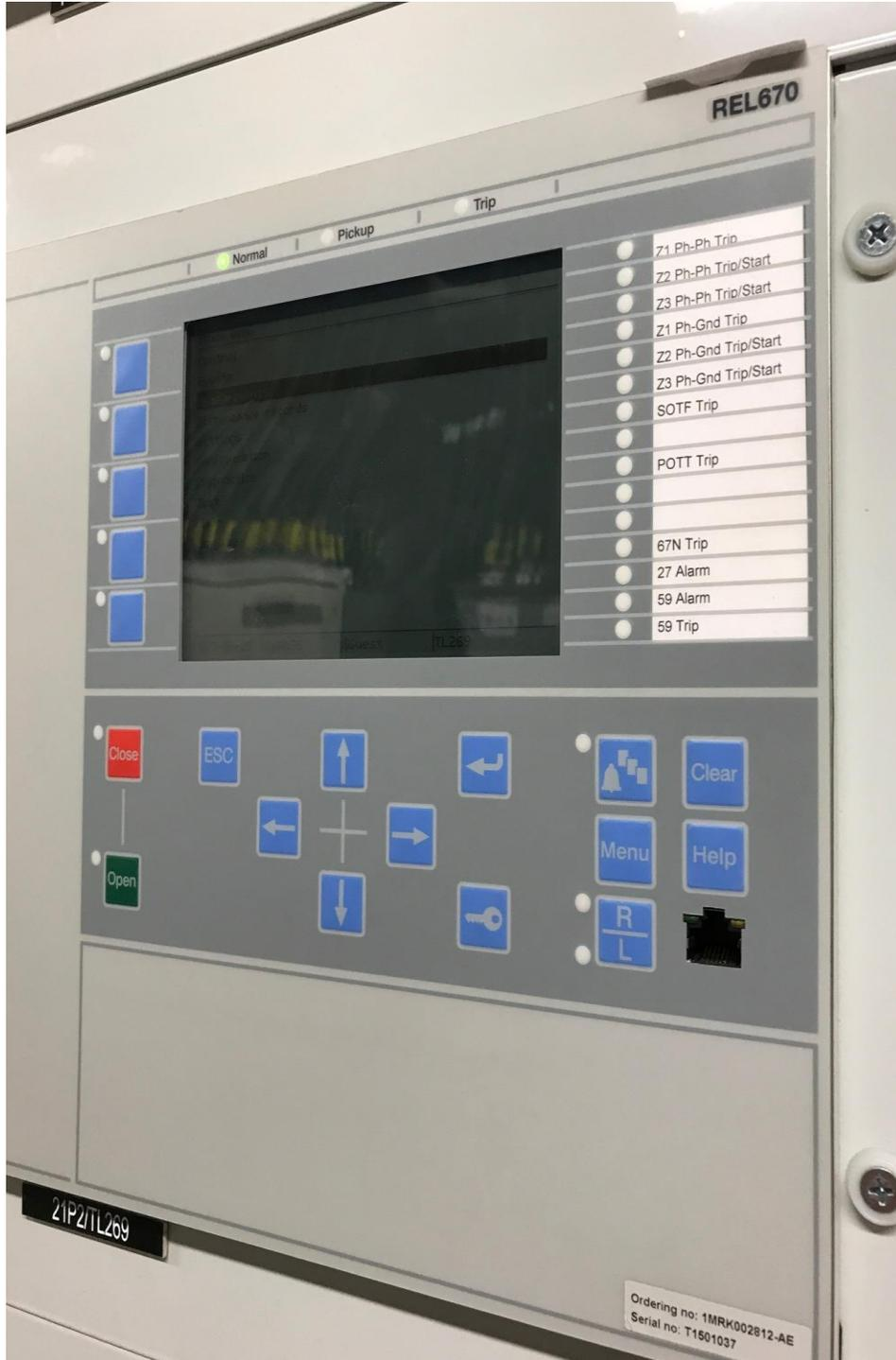
**Photo 2:** 230kV AC Line Protection Relay.
