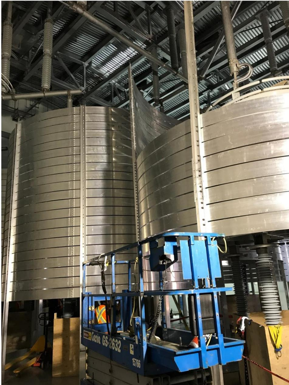
**Photo 7:** Converter Station – DC reactors shielding installation.
