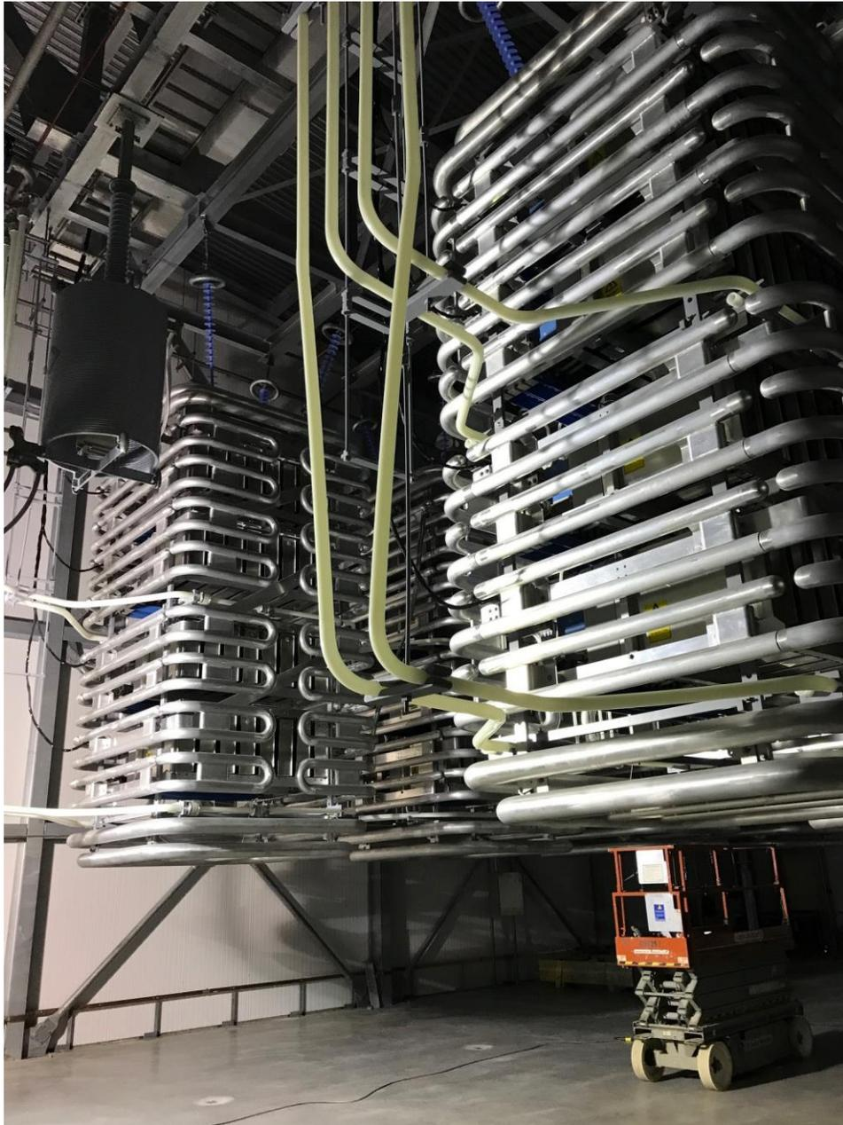
**Photo 6:** Converter Station – HVdc valves with cooling piping installed.
