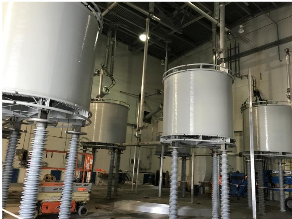
**Photo 16:** Converter Station – Reactor hall (DC reactors). Shielding is yet to be installed.
