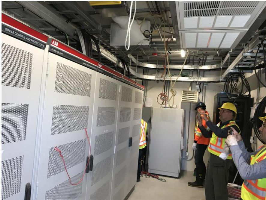
**Photo 14:** Point Aconi Transition Compound – P&C cabinets installed in the control room.
