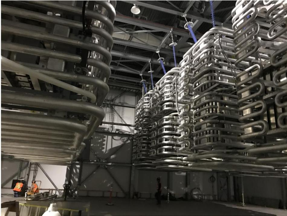
**Photo 15:** Converter Station – HVdc valves with shields and cooling piping installed.
