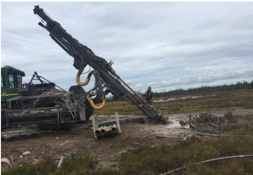
**Photo 8:** HVDC – Anchor drilling.
