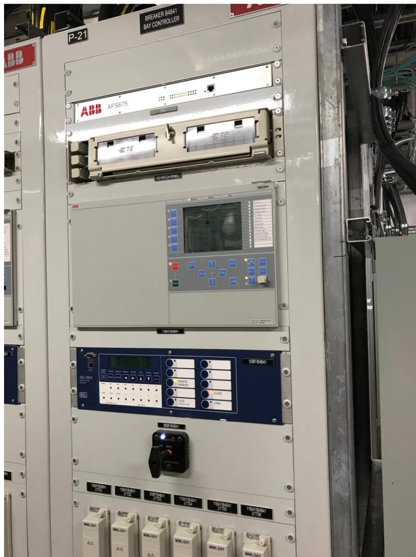
**Photo 1:** AC circuit breaker controller.
