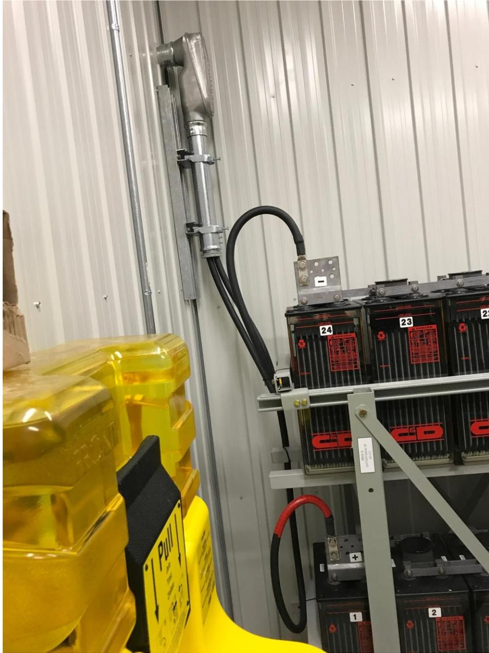
**Photo 3:** 125Vdc Station Battery termination.
