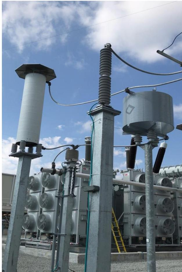
**Photo 16:** Converter Station AC Yard – converter transformer with resistor(left) and reactor (right).
