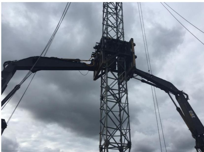
**Photo 9:** HVDC – Holding the tower while the crew is working on the 4 anchors.
