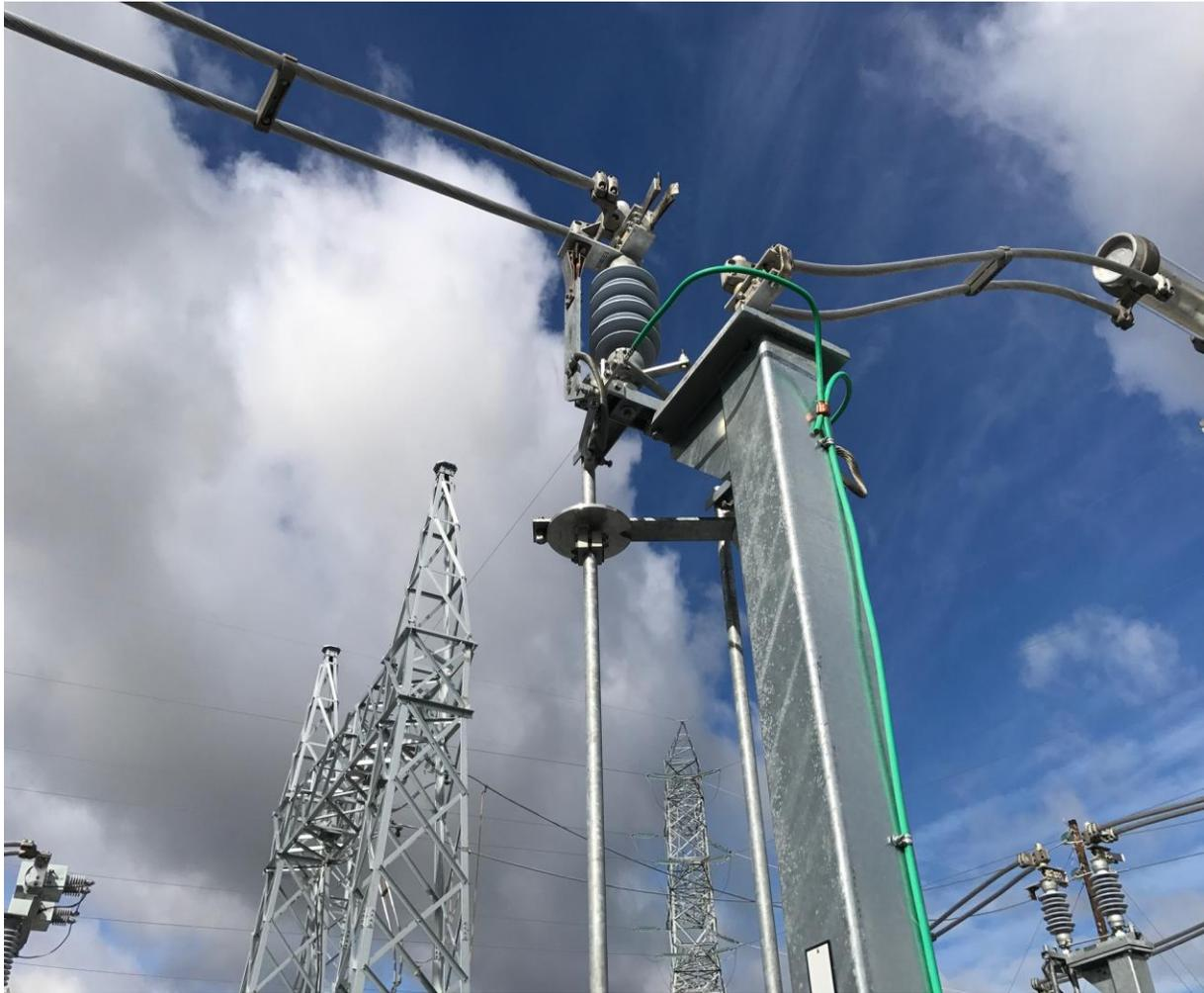
**Photo 5:** DC Neutral grounding switch detail.
