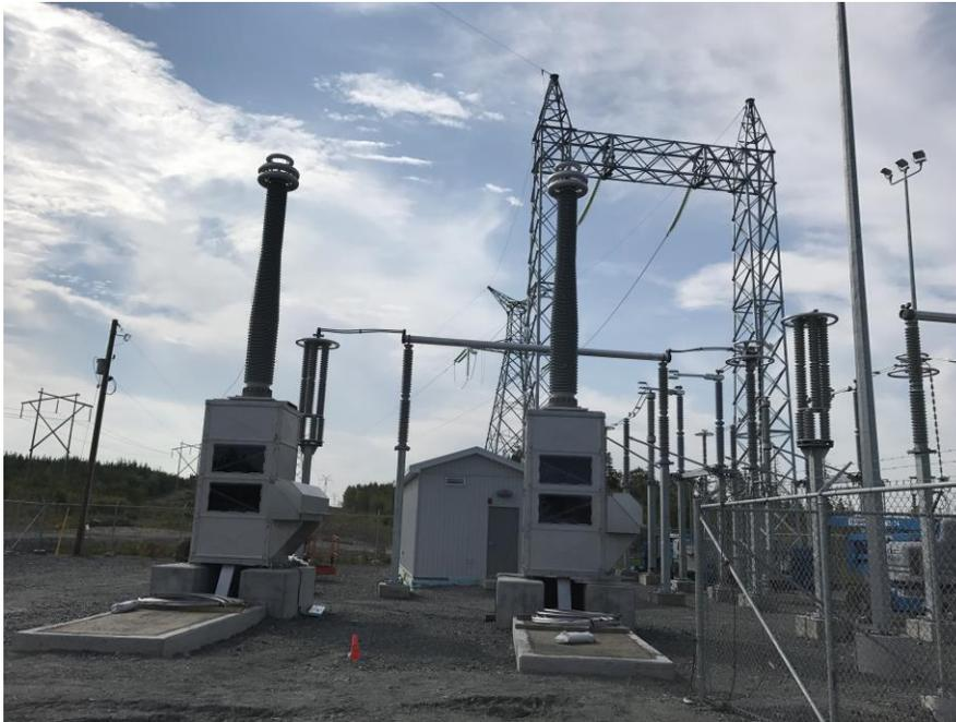
**Photo 13:** Point Aconi Transition Compound – land cables terminations with control room, gantry and HVdc tower on the background.
